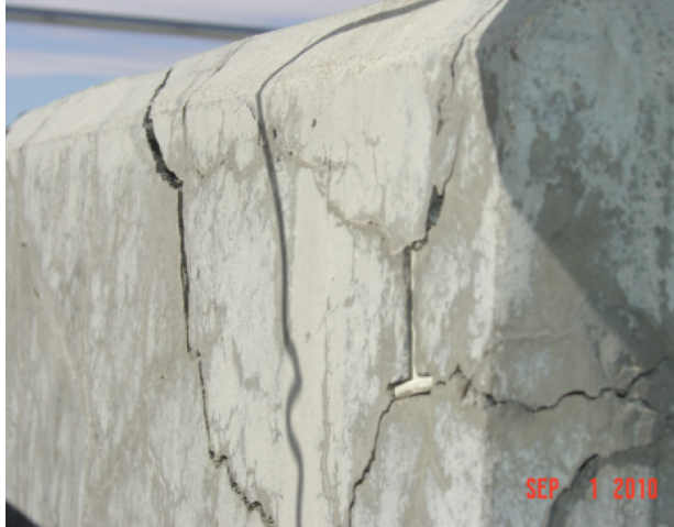
Figure 2-2. Photograph of Cracks on the Corner of a Horizontal Storage Module, Prior to Repair, at the Three Mile Island, Unit 2 Spent Fuel Storage Facility at Idaho National Laboratory (NRC, 2012)
