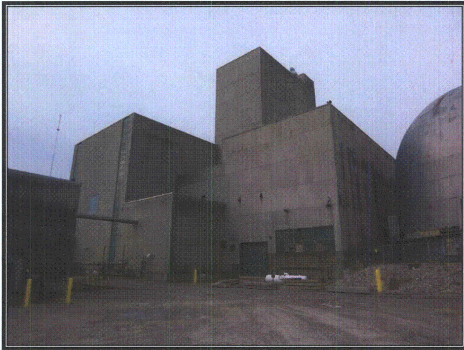
Plate 48 Steam generator building looking southwest (Photograph by RCG&A, 2008)
