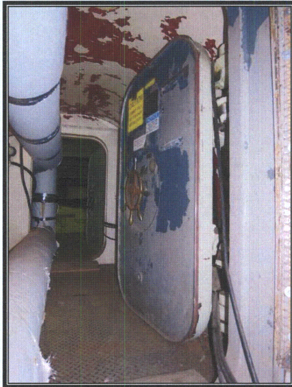
Plate 62 Outer personnel access door (Photograph by RCG&A, 2008)
