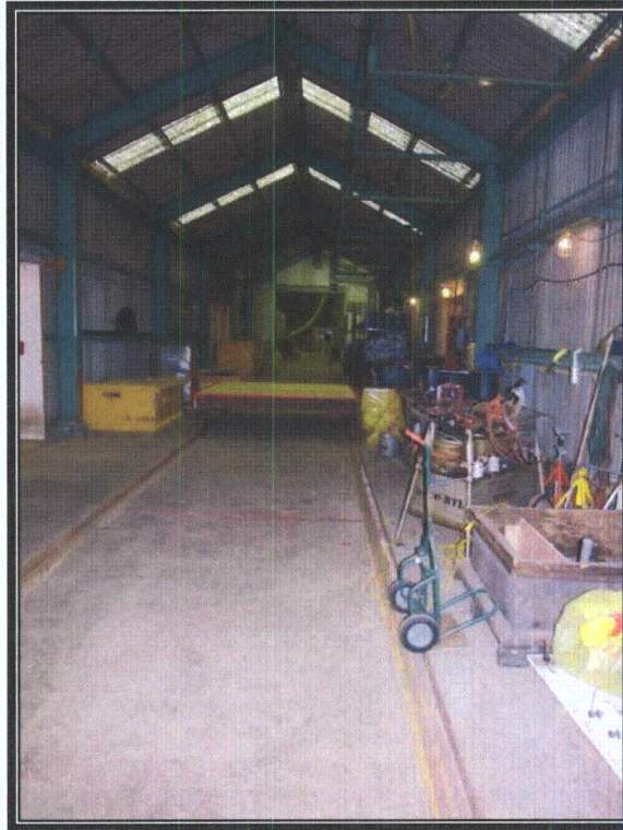
Plate 97 Interior of trestleway looking north (Photograph by RCG&A, 2008)
