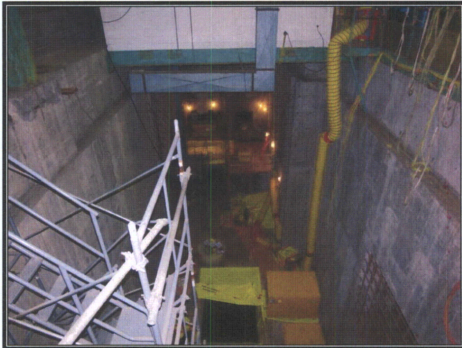
Plate 114 Equipment repair pit (Photograph by RCG&A, 2008)
