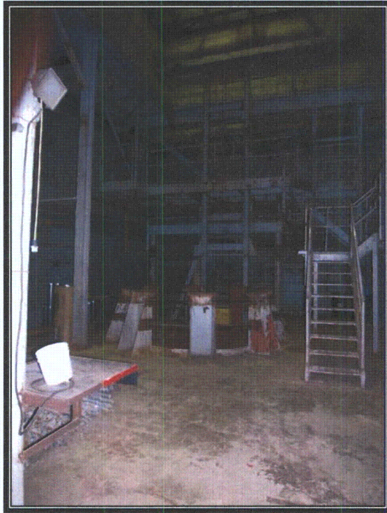
Plate 54 Mounting location for steam generator (Photograph by RCG&A, 2008)
