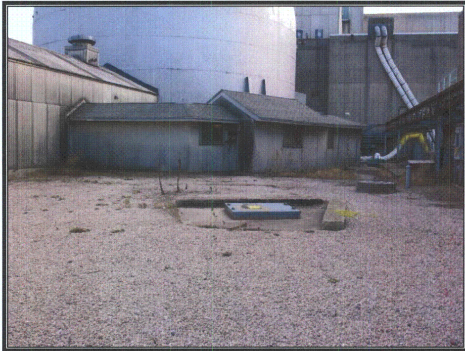
Plate 64 Building connecting outer personnel door to trestleway (Photograph by RCG&A, 2008)
