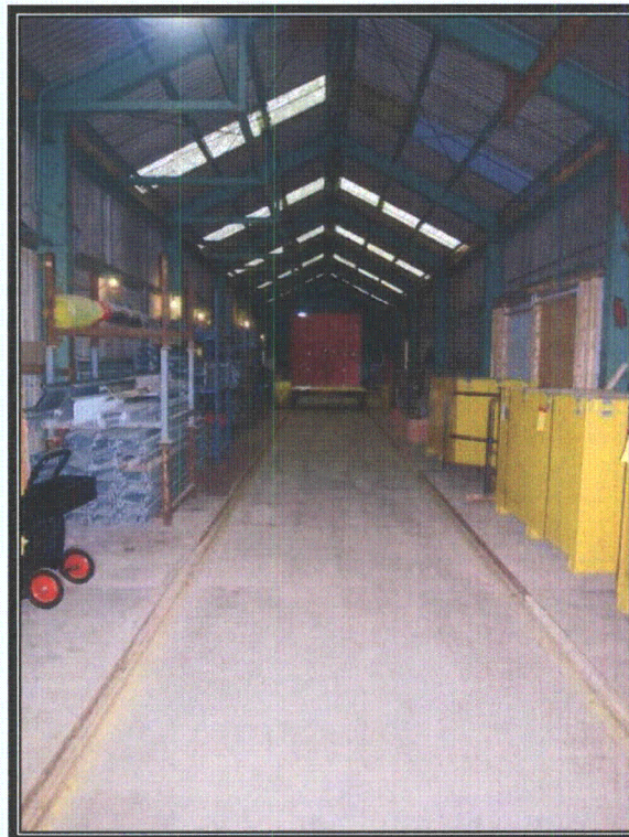
Plate 98 Interior of trestleway looking south, toward reactor building (Photograph by RCG&A, 2008)
