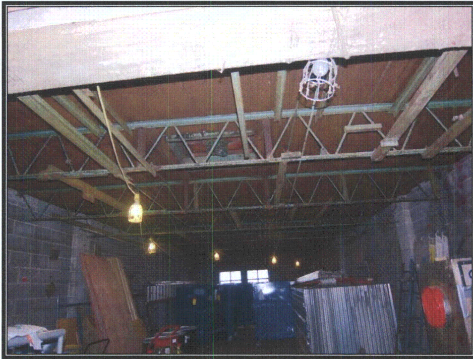
Plate 105 Vent building roof detail (Photograph by RCG&A, 2008)
