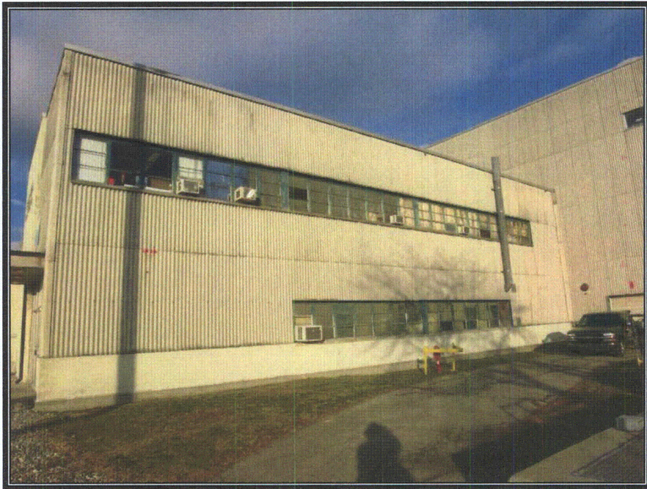
Plate 46 South wall of office building (Photograph by RCG&A, 2008)
