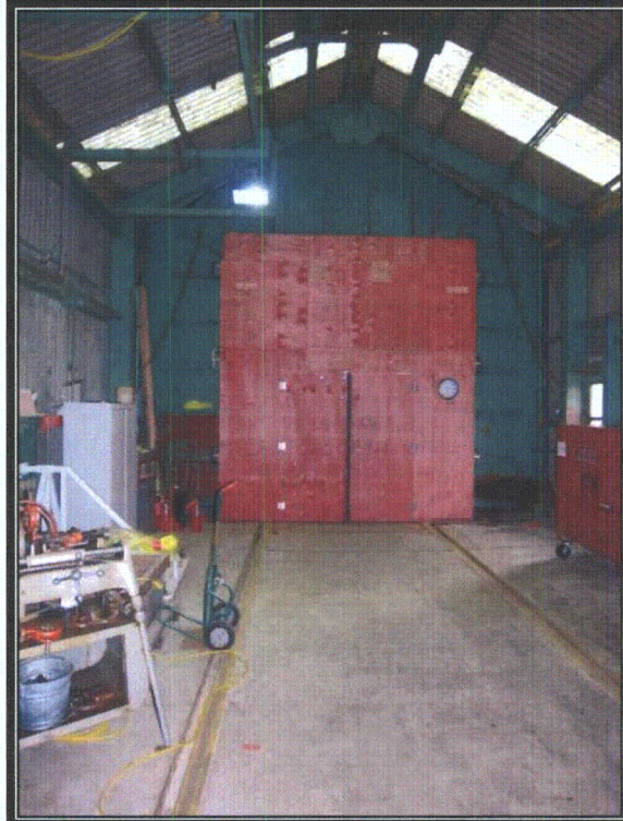
Plate 100 View looking south showing cask car rails (Photograph by RCG&A, 2008)
