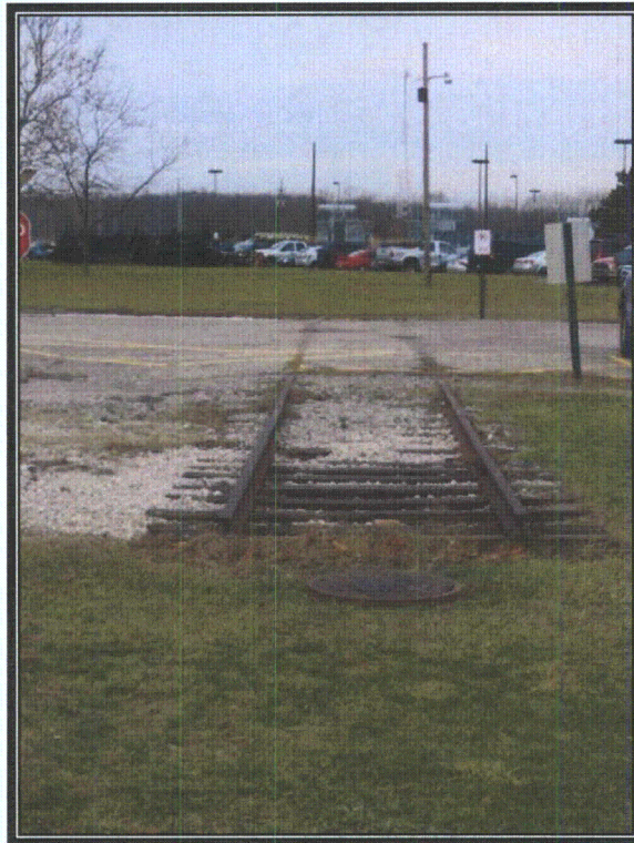
Plate 23 Abandoned railroad tracks west of turbine building (Photograph by RCG&A, 2008)
