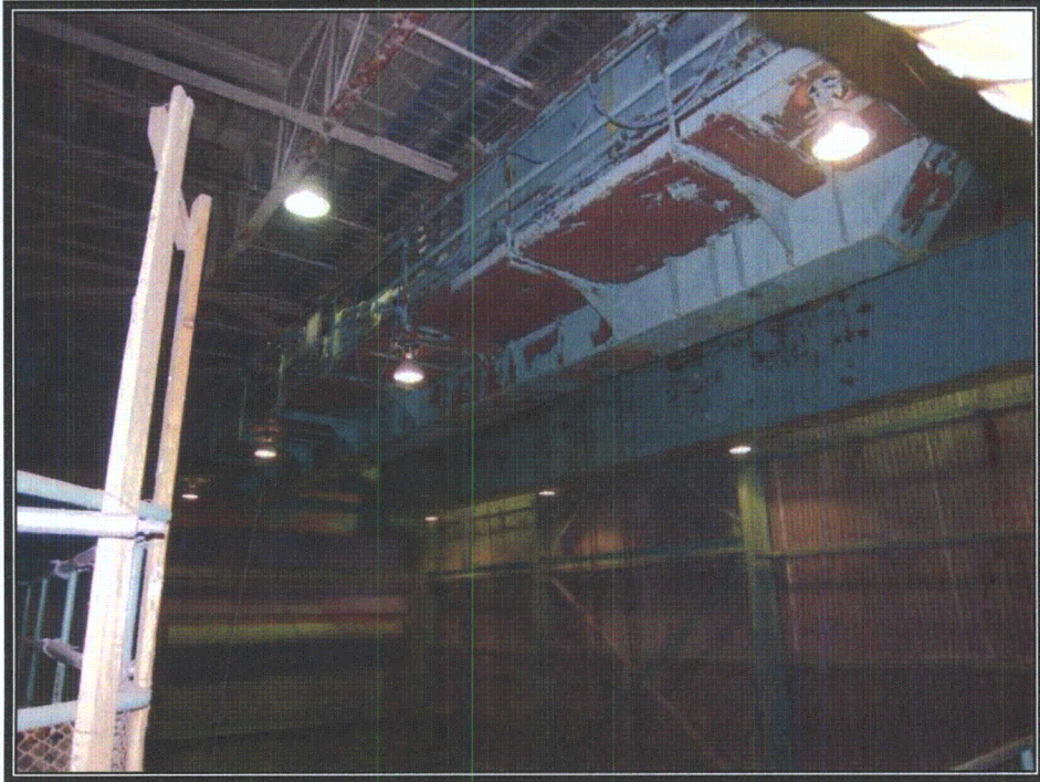
Plate 107 Interior of FARB looking northwest (Photograph by RCG&A, 2008)
