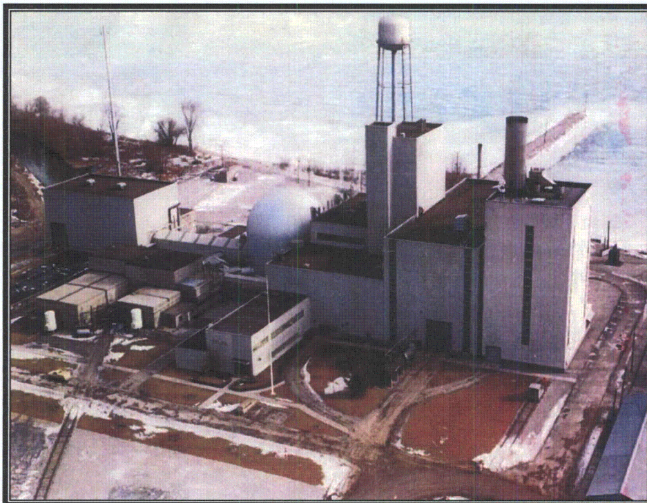
Plate 41 Aerial view of plant showing boiler house to the right, ca. 1975 (Courtesy DECo)
