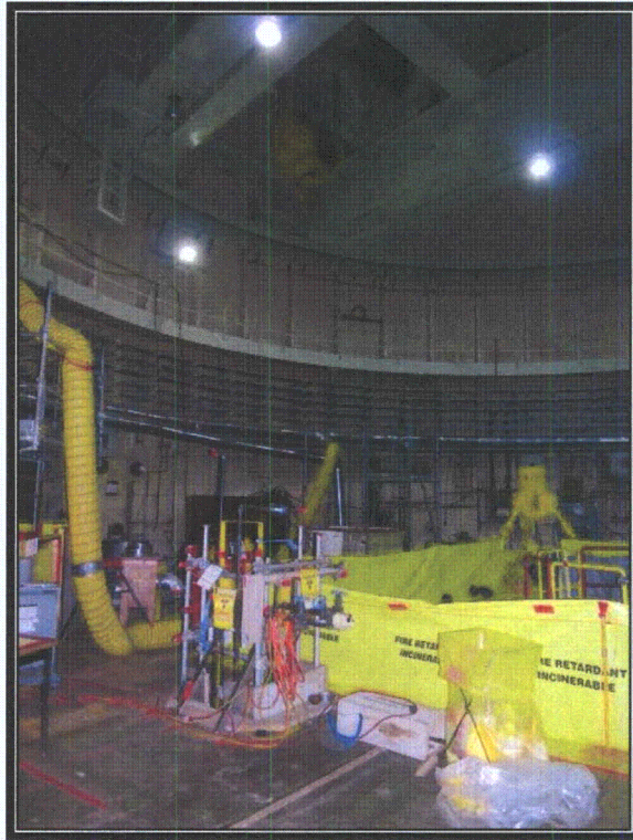
Plate 38 Interior of reactor building, note bracket on wall for television camera (Photograph by RCG&A, 2008)
