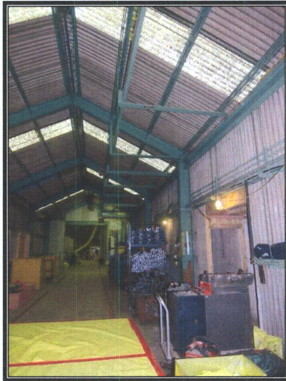
Plate 99 Extension at top of wall for electric cables (Photograph by RCG&A, 2008)
