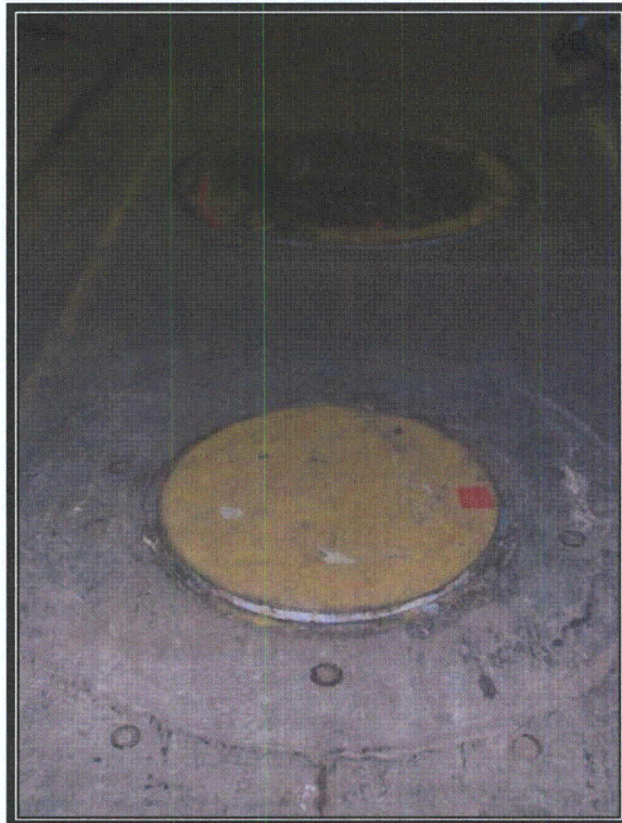
Plate 122 Transfer tank entrance port (Photograph by RCG&A, 2008)
