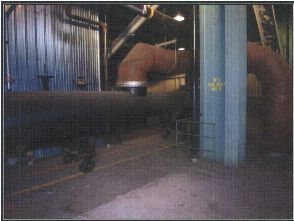
Plate 30 Feedwater heater on turbine level (Photograph by RCG&A, 2008)
