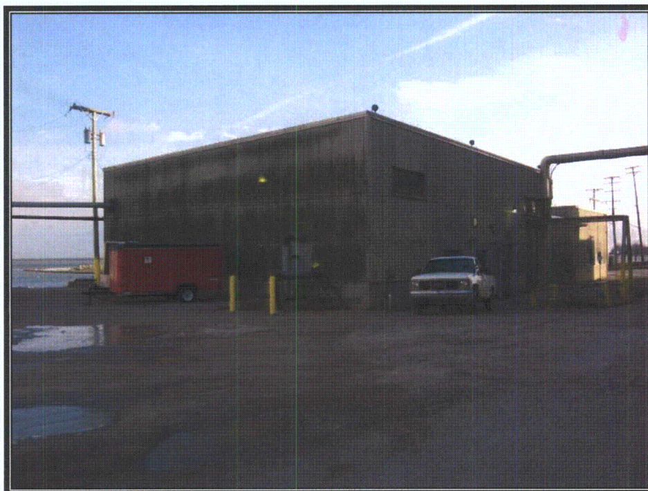
Plate 146 View of plant services building looking southeast (Photograph by RCG&A, 2008)
