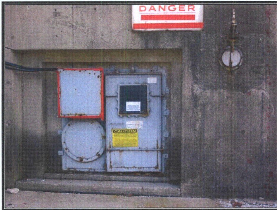
Plate 142 Access portal to building (Photograph by RCG&A, 2008)
