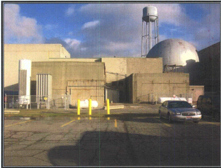
Plate 135 View of sodium service building looking east (Photograph by RCG&A, 2008)
