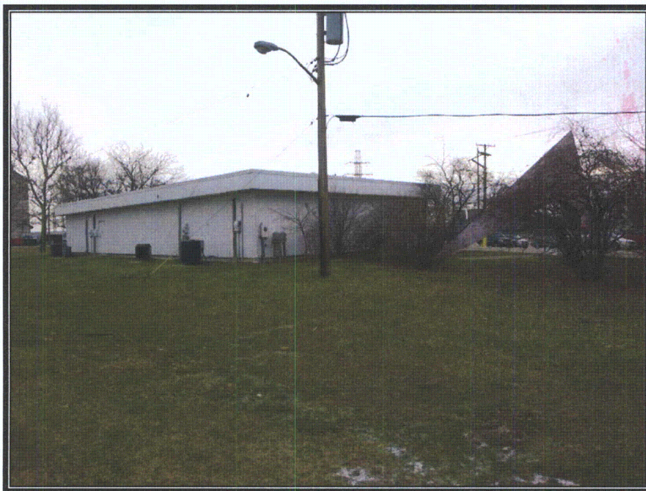
Plate 149 View of visitor's center looking east (Photograph by RCG&A, 2008)
