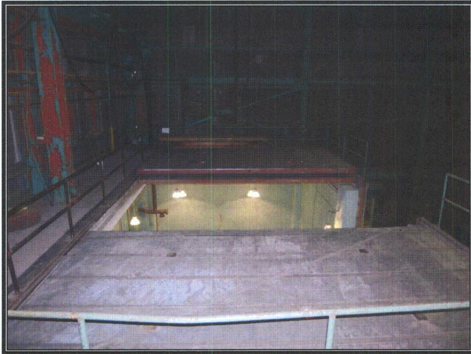
Plate 125 Removable roof section of cut-off pool roof (Photograph by RCG&A, 2008)
