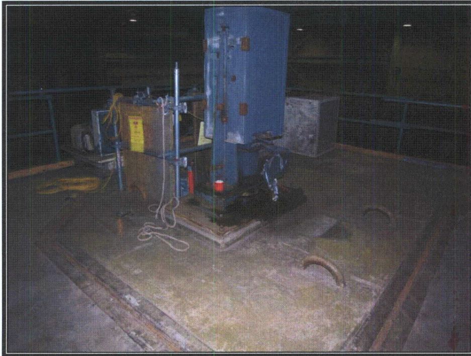
Plate 127 Removable roof section of steam cleaning chamber (Photograph by RCG&A, 2008)
