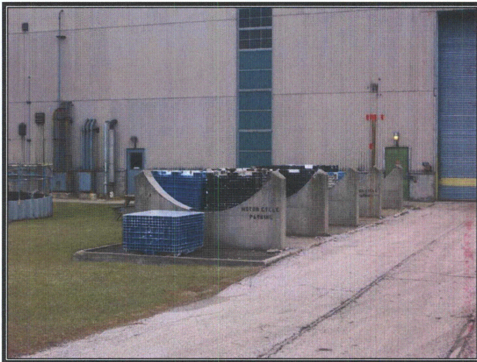
Plate 151 Concrete tank saddles (Photograph by RCG&A, 2008)
