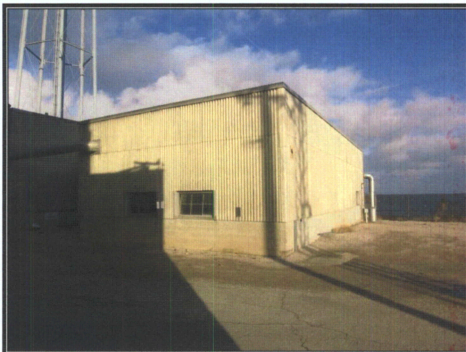
Plate 145 View of screen house looking northeast (Photograph by RCG&A, 2008)
