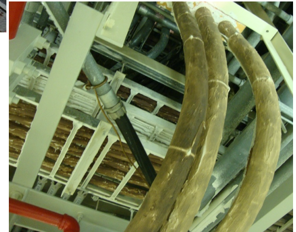
Cable coatings showing change from their original white color.
