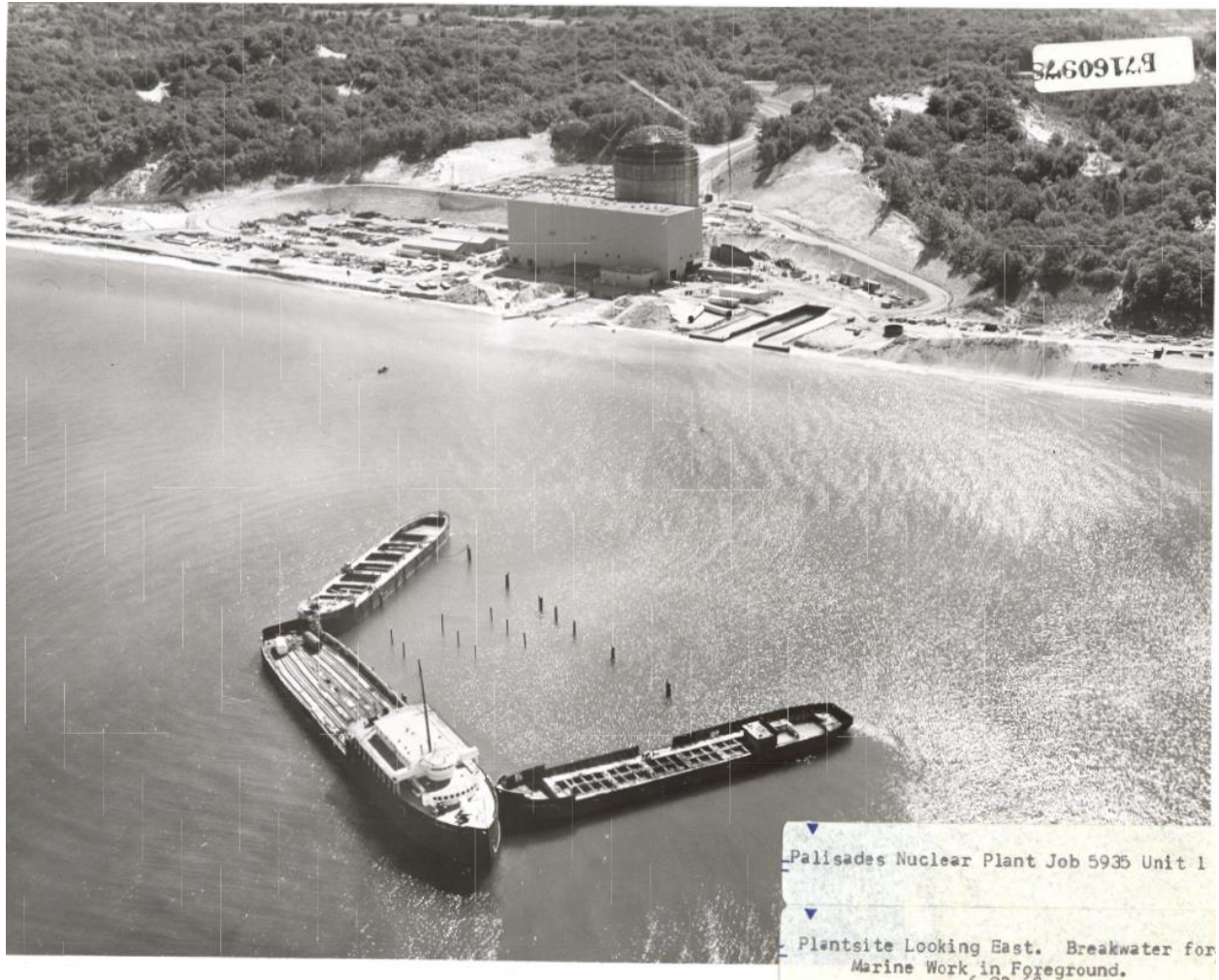
Figure I-11 A Photograph from June 1968, Looking East over the Palisades Nuclear Plant Site. Note the Cleared Vegetation and Road Cut into the Sand Dune to the Right of the Reactor Vessel Building and the Land Grading and Vegetation Clearing along the Beach to the South of the Site. Source: HDI 2024-TN10670.
