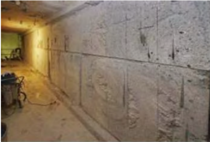
Shaved walls after decontamination
