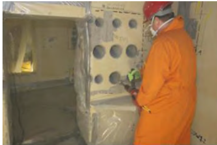
Drill out of ducts and wire shafts
