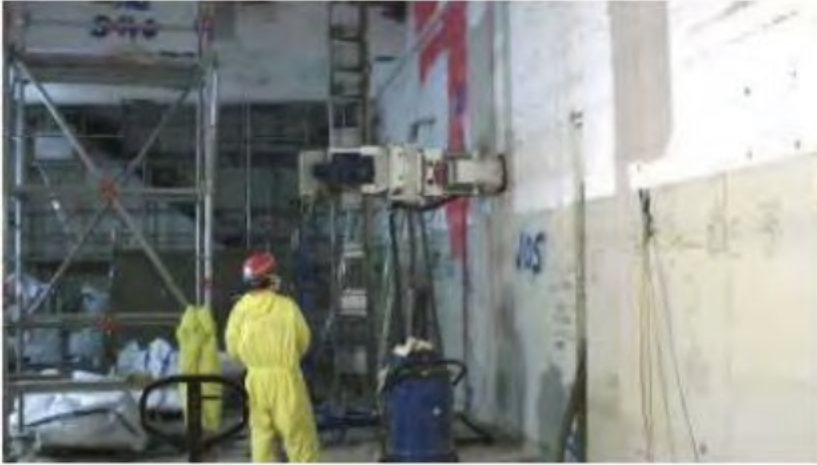
Wall decontamination
