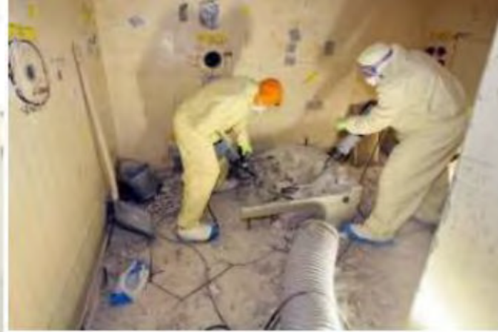
Electric handhold chiseling
