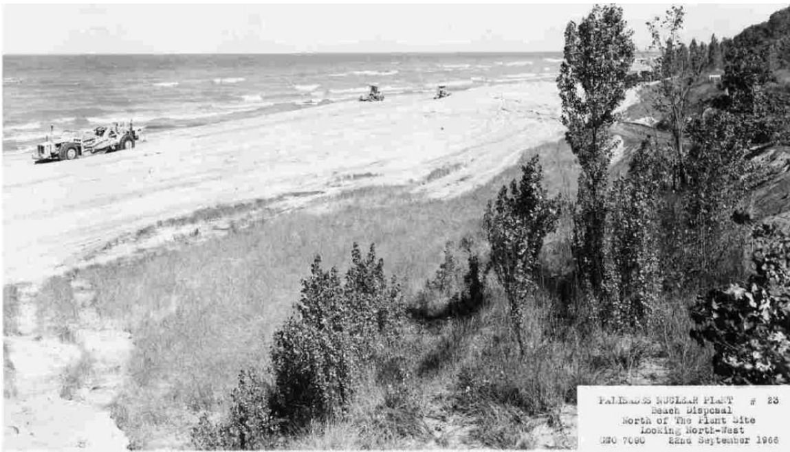
Figure I-4 Heavy Equipment Operating on the Beach on the Northern Portion of the Palisades Nuclear Plant Site on September 22, 1966. Photograph Looking to the Northwest. Source: HDI 2024-TN10670.
