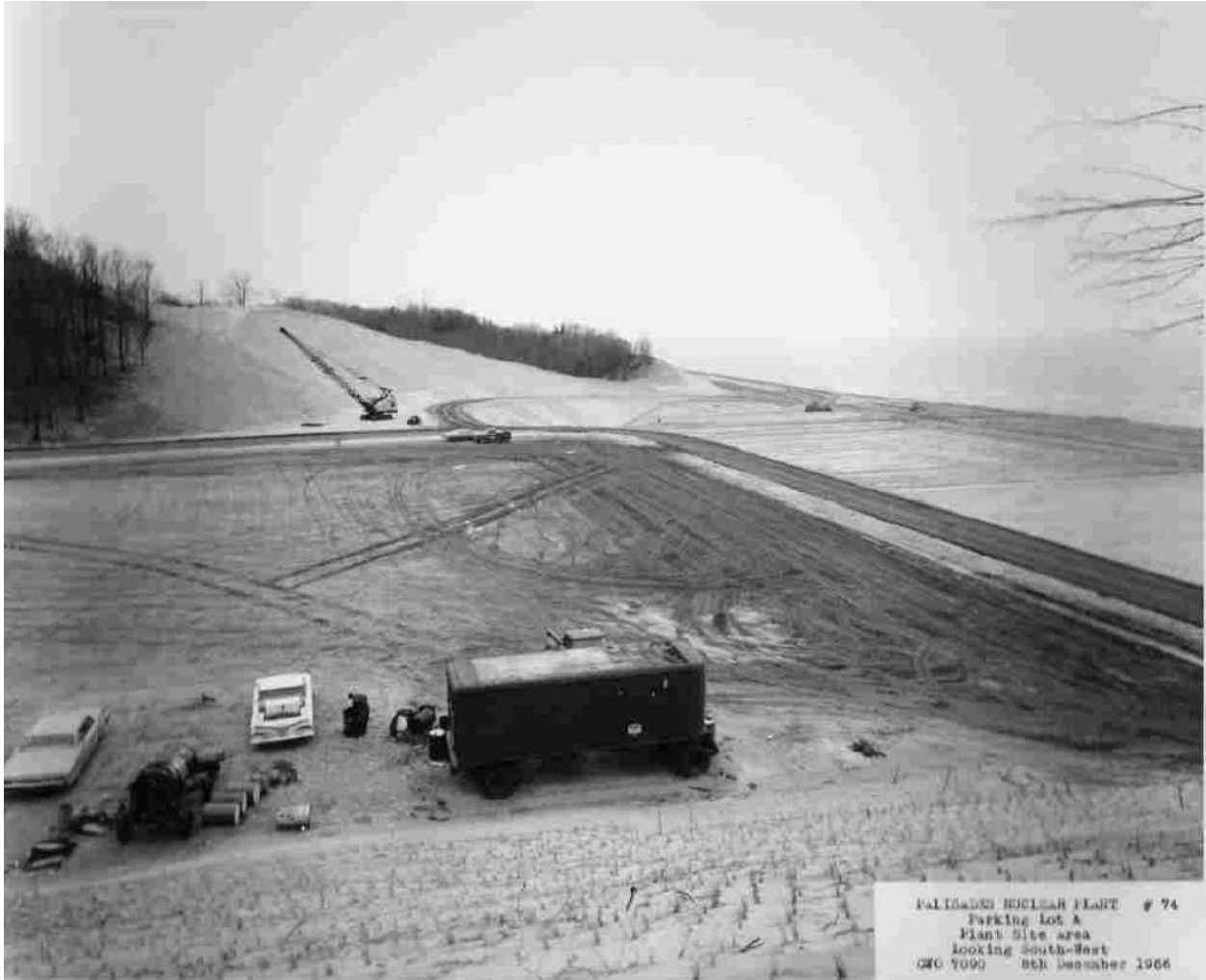
Figure I-6 A Photograph from December 1966 Looking Southwest across the Palisades Nuclear Plant Site Showing the Extent of Land Grading Activities at That Time. Note the Cleared Vegetation and Road Cut into the Sand Dune behind the Crane. Source: HDI 2024-TN10670.
