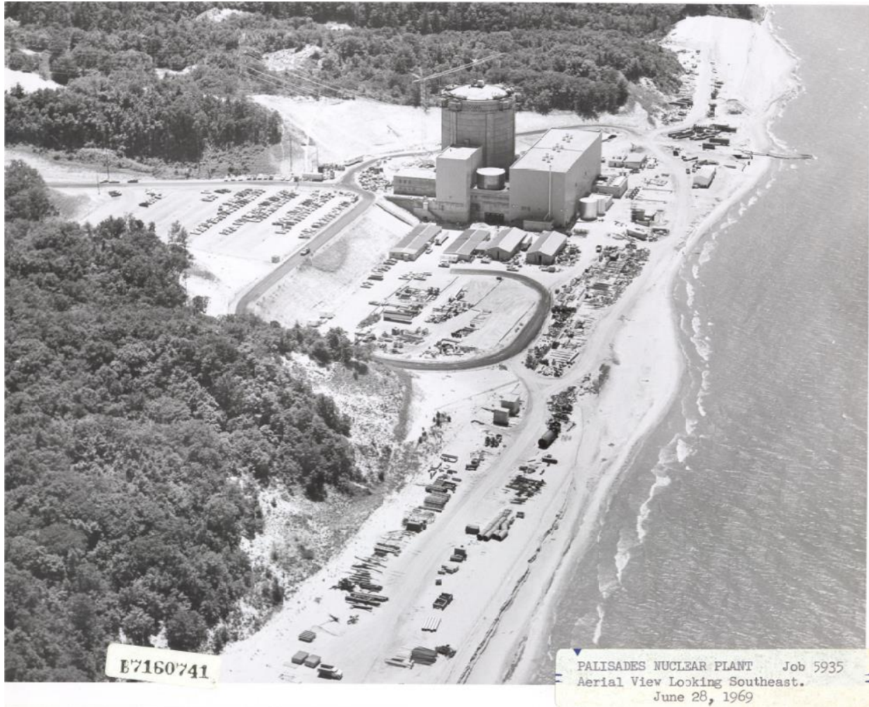
Figure I-16 A Photograph from June 28, 1969, Looking South over Palisades Nuclear Plant Site. Note the Cleared Vegetation and Road Cut into the Sand Dune to the Left of the Reactor Vessel Building and the Land Grading and Vegetation Clearing along the Beach to the South of the Site. This Location Is Where Both Cooling Towers Exist Today. Source: HDI 2024-TN10670.
