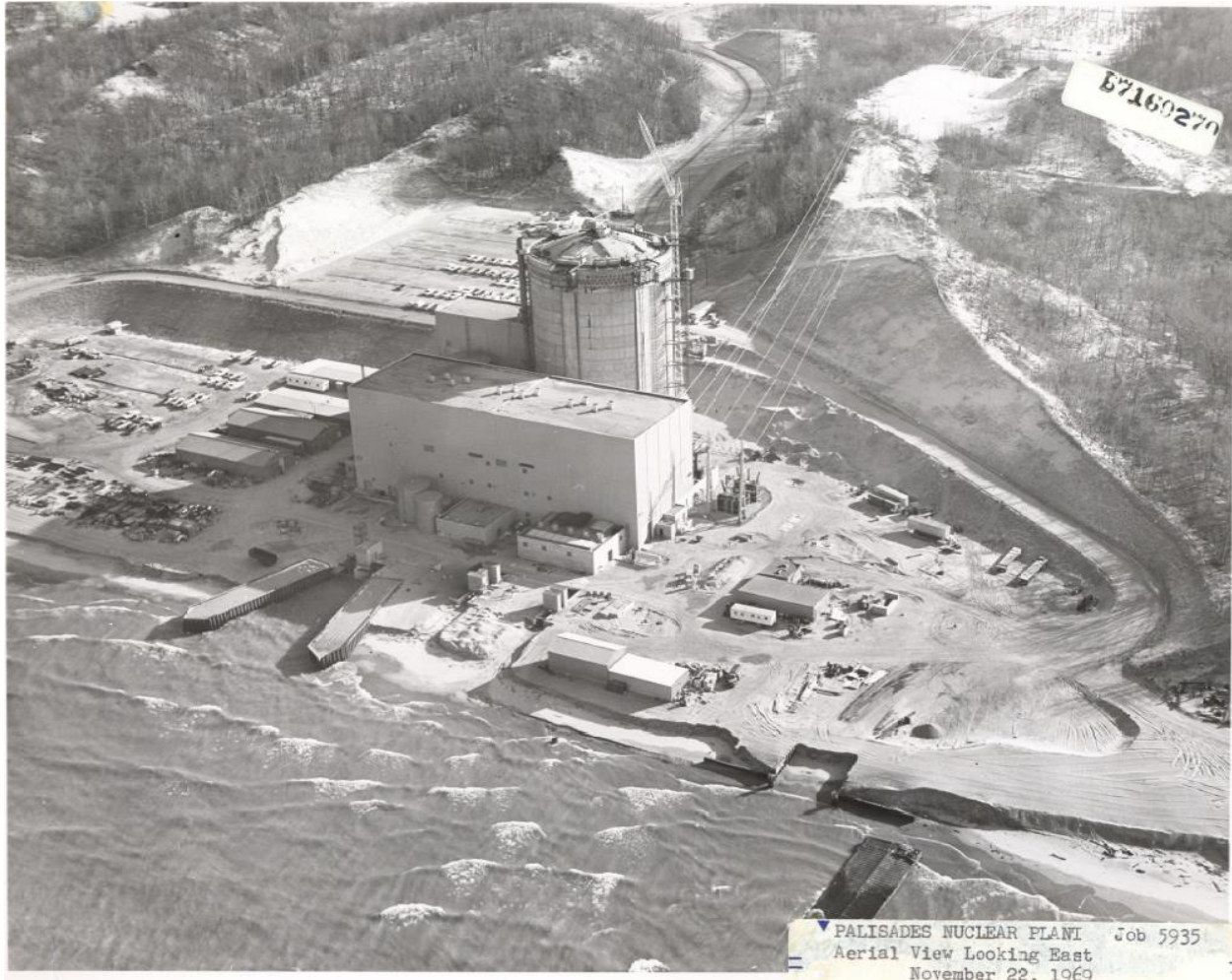
Figure I-17 A Photograph from November 22, 1969, Looking Northeast over the Palisades Nuclear Plant Site. Note the Cleared Vegetation and Road Cut into the Sand Dune to the Right of the Reactor Vessel Building and the Land Grading and Vegetation Clearing along the Beach to the South of the Site. Source: HDI 2024-TN10670.
