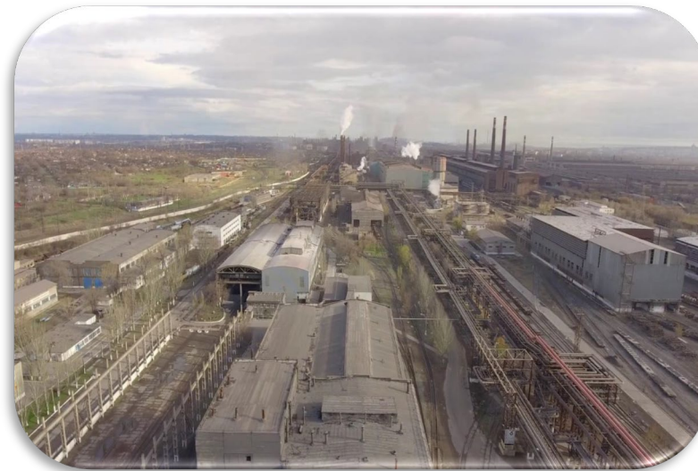
Integrated Steel Manufacturing Plant
