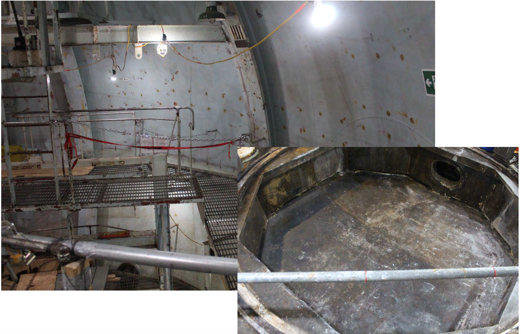
Containment Vessel – After
