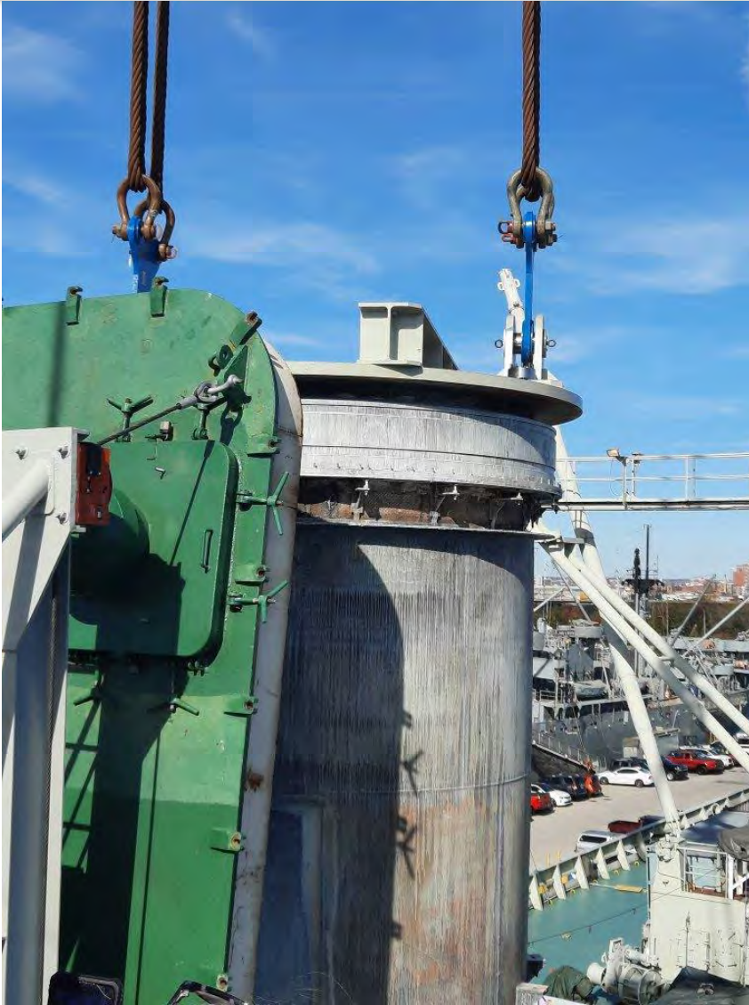
N.S. SAVANNAH Reactor Vessel removal, November 8, 2022
