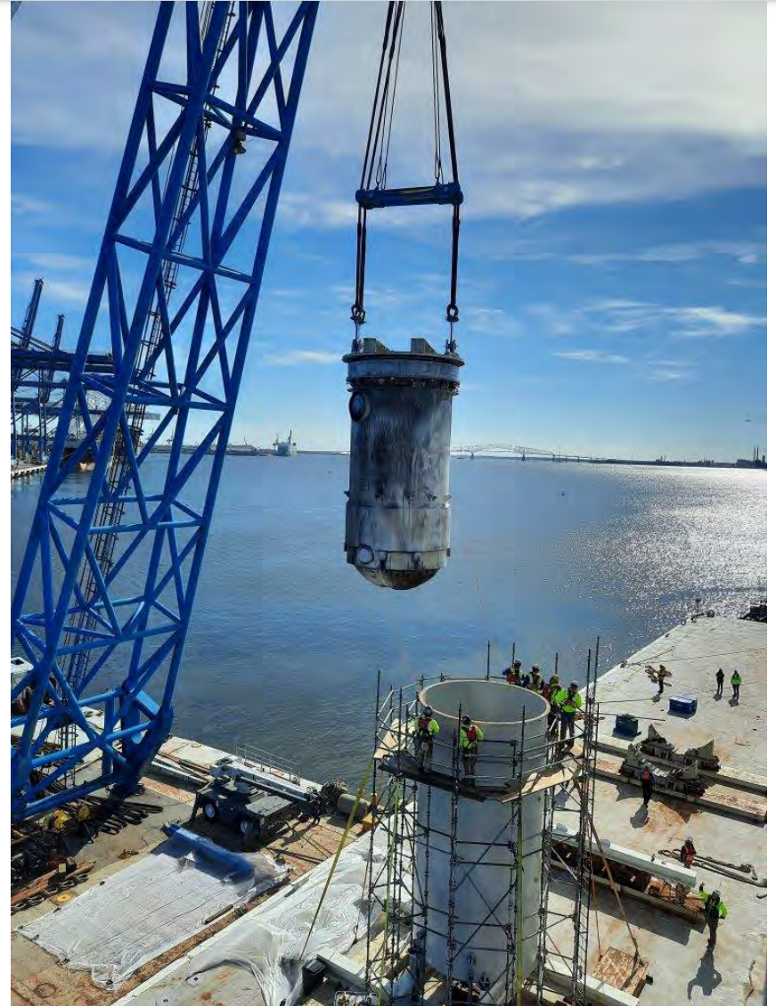
N.S. SAVANNAH Reactor Vessel removal, November 8, 2022
