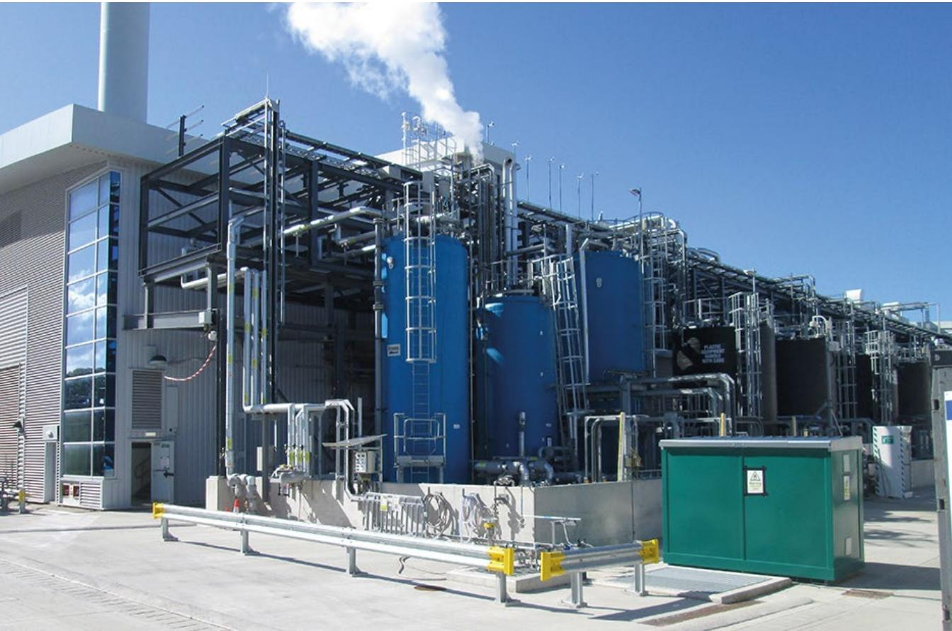
The Tails Management Facility manages deconversion of depleted Uranium Hexafluoride ( $UF_6$ ) – to stable Uranium Oxide ( $U_3O_8$ ) and Hydrofluoric Acid (HF).
