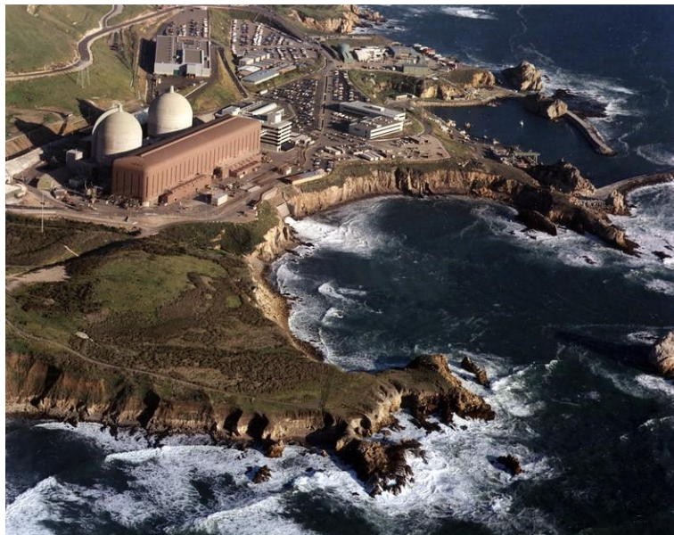
Diablo Canyon Nuclear Power Plant, Units 1 and 2, Avila Beach, California (Source: Photo courtesy of ©Pacific Gas and Electric)
