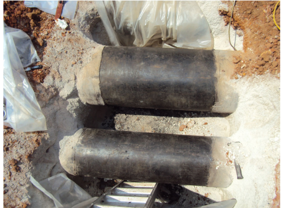
Residual Heat Removal Service Water Pipe (Top) and Emergency Equipment Cooling Water Pipe (Bottom) June 2010 – Coating Removed
