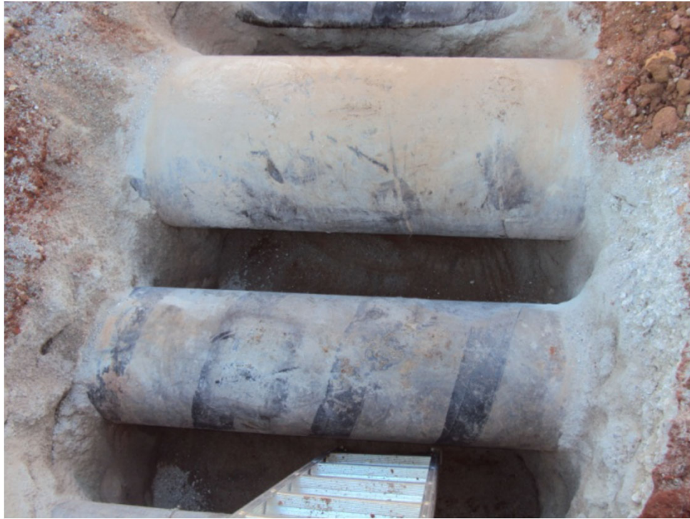
Residual Heat Removal Service Water Pipe (Top) and Emergency Equipment Cooling Water Pipe (Bottom) June 2010 – Prior to Coating Removal
