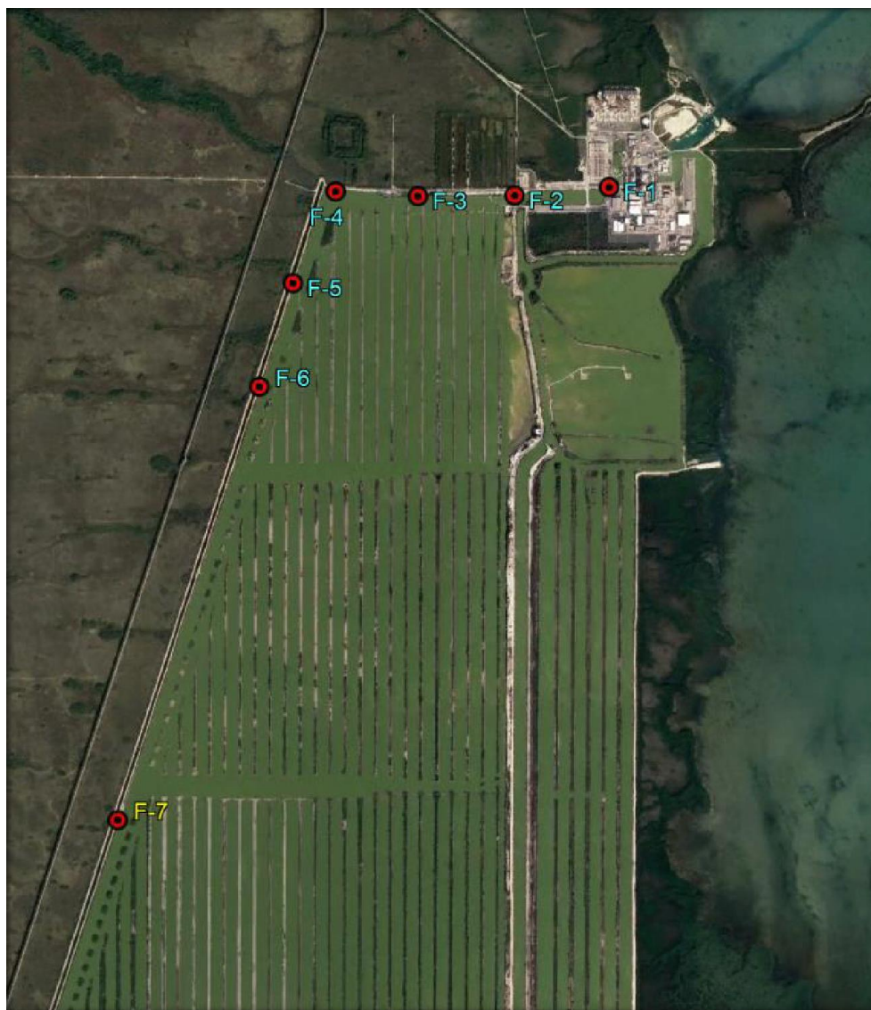
Figure 2-2 FPL Freshening Well Locations (Source: FPL 2020a)
