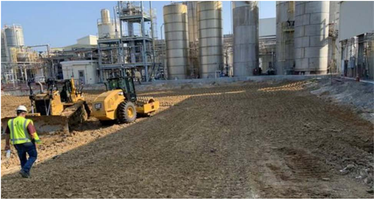
Figure 7 – Backfill and Compaction Process
