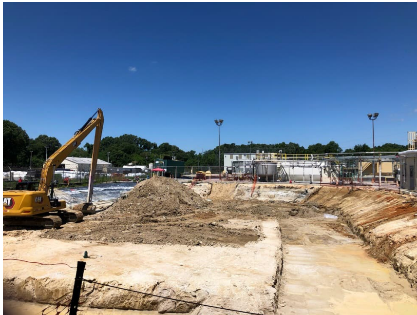
Figure 6 – Sub-Liner Soil Excavation
