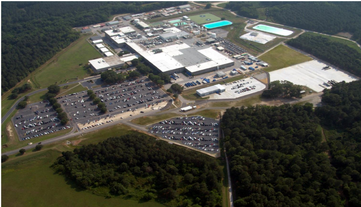
Figure 3-23 Aerial View of the CFFF Site and Facilities (WEC 2012-TN6697)
