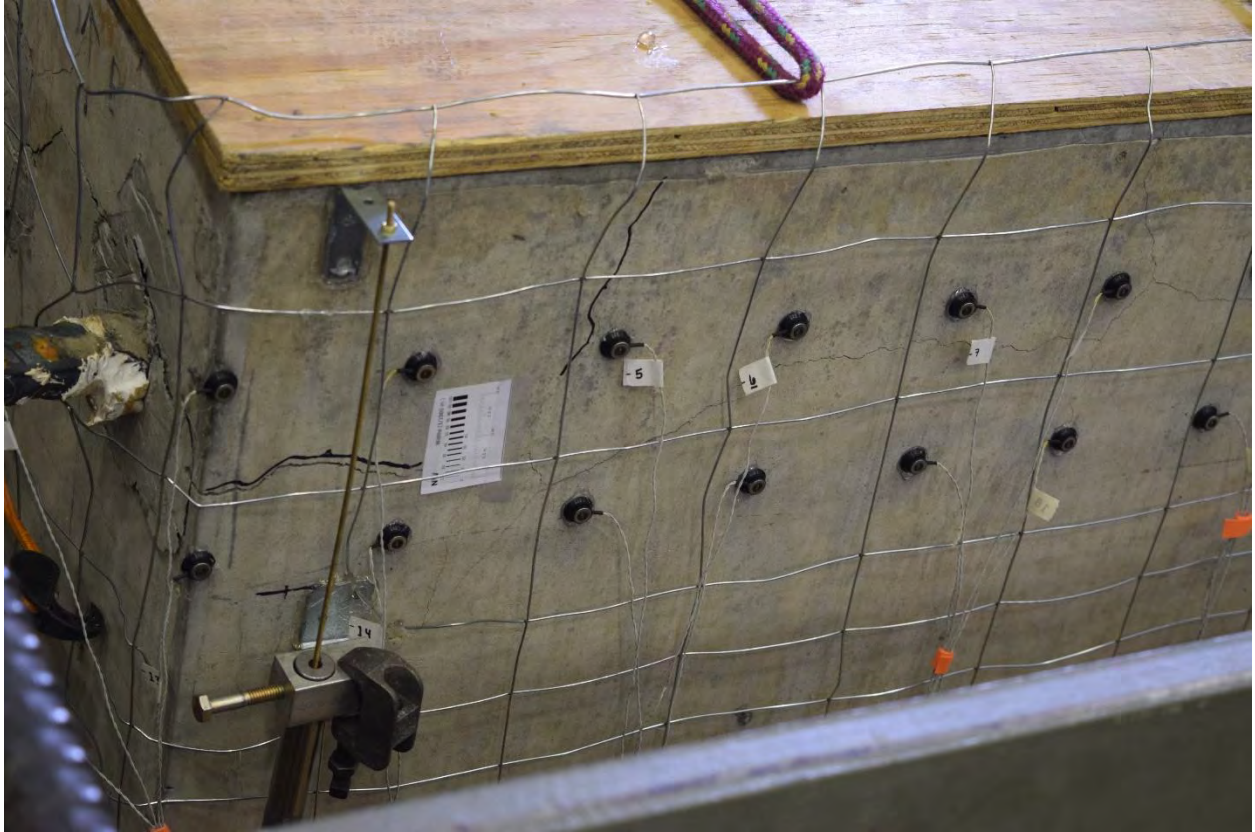
Figure 84 Test Photo Specimen D3, NW corner, 108 kips
