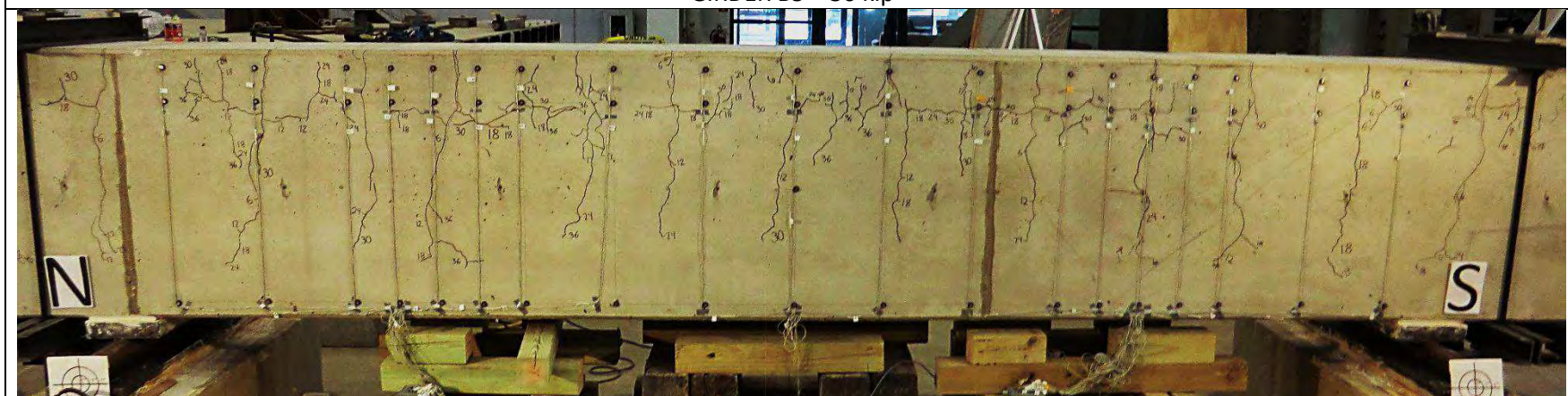
GIRDER B6 – 1 kip
