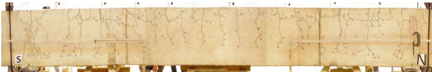
Figure 10 East Elevation of Test Girder A4 Reloaded to 36 kip
