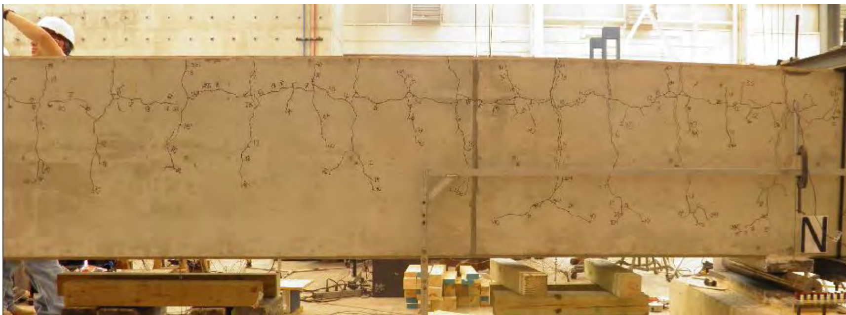
Figure 6 Flexural Cracks and Bursting Cracks
