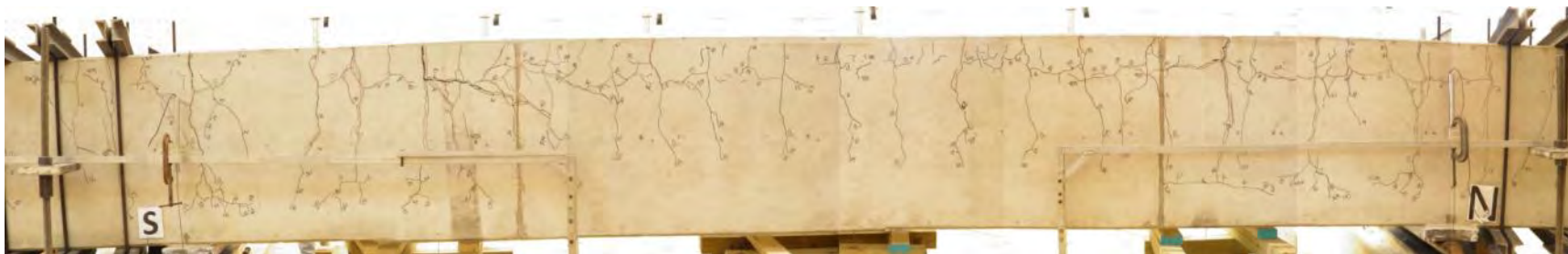
Figure 12 East Elevation of Test Girder A4 Reloaded to 42 kip
