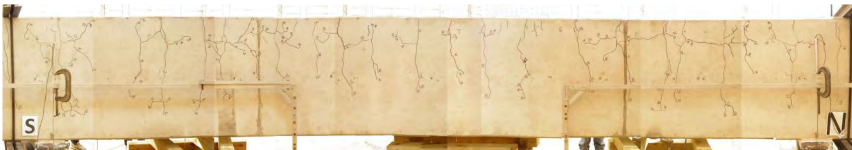
Figure 8 East Elevation of Test Girder A4. Initial Loading. Applied Load = 36 kip
