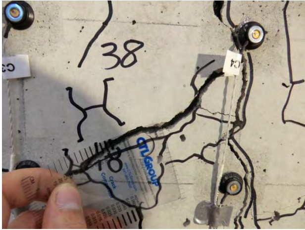
Girder A-1, Load = 36 kip (reload).
