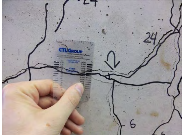
Girder B-2, Load = 36 kip (reload).
