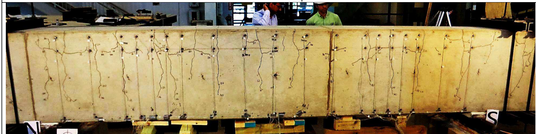
GIRDER B4 – 36 kip
