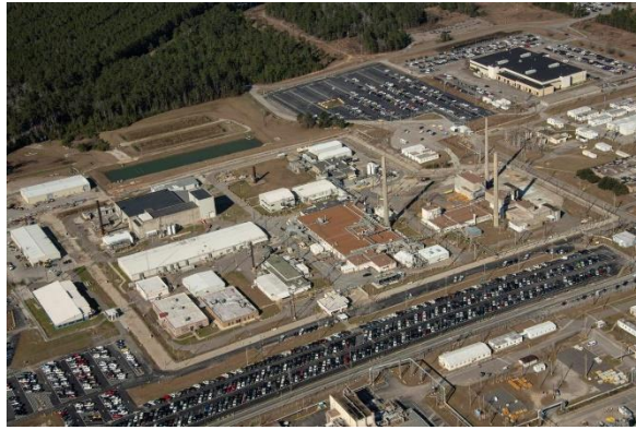
Tritium complex in H-Area at the Savannah River Site. DOE photo.
