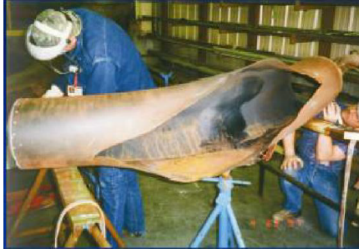
Figure 3-9 Ruptured elbow caused by FAC. (Ahmed 2012)
