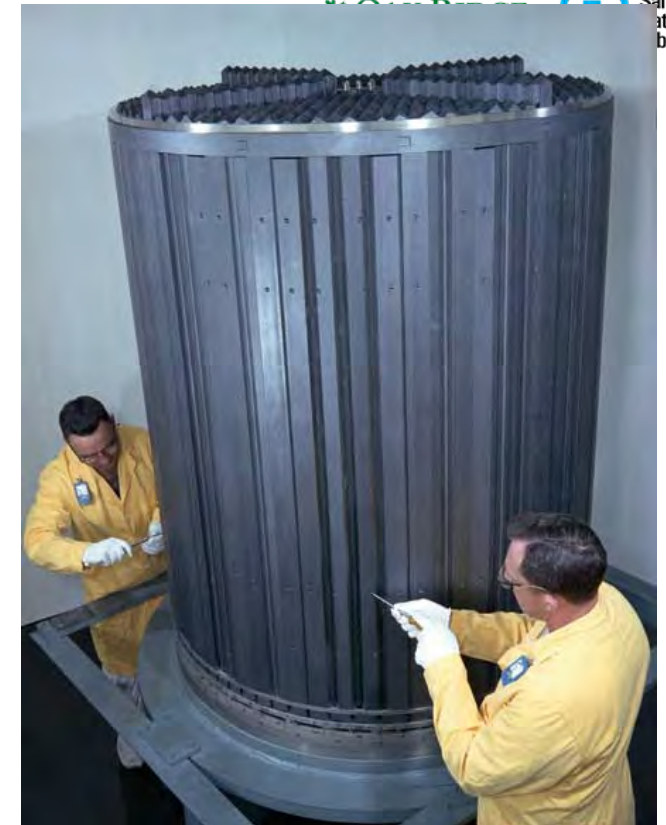
MSRE Graphite Core Structure [ https://en.wikipedia.org/wiki/Molten-Salt_Reactor_Experiment ]
