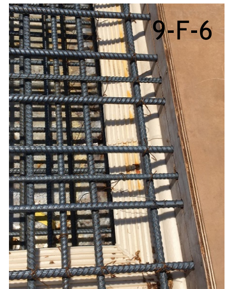
Embedded Floor Water Stop
