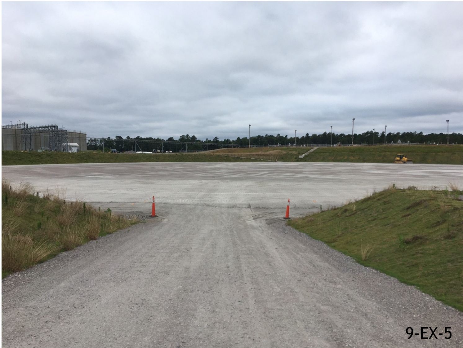
Southeast corner looking northwest
