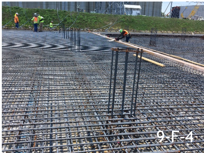
Column Reinforcing Bar
