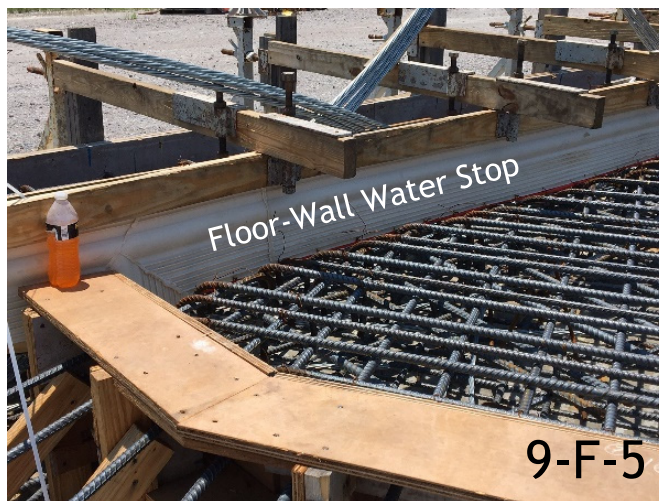
Exterior Floor Forming
