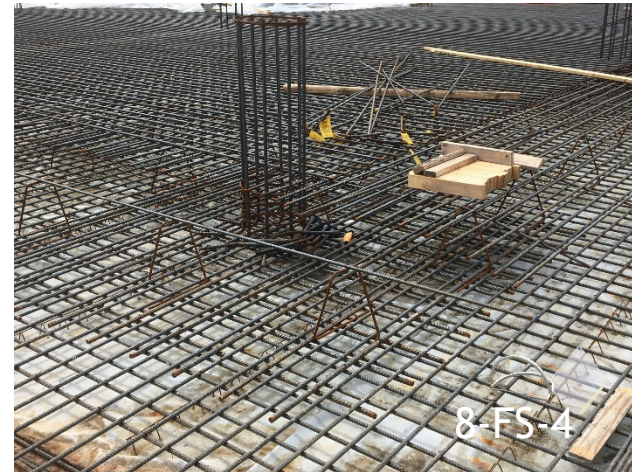
Floor/ Column Rebar
