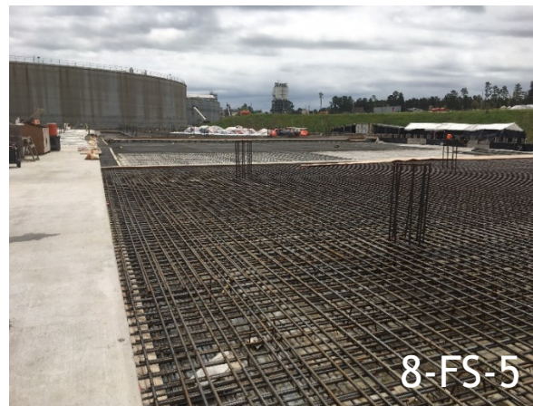
Floor Section Ready for Concrete
