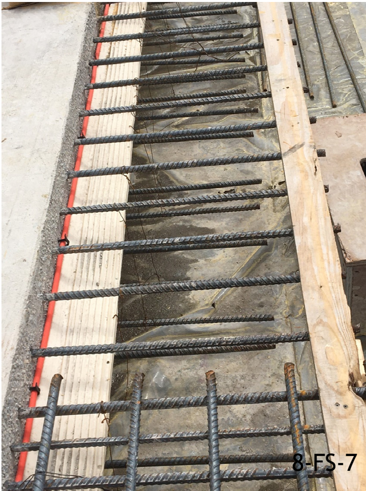
Floor Section with Embedded Water stop
