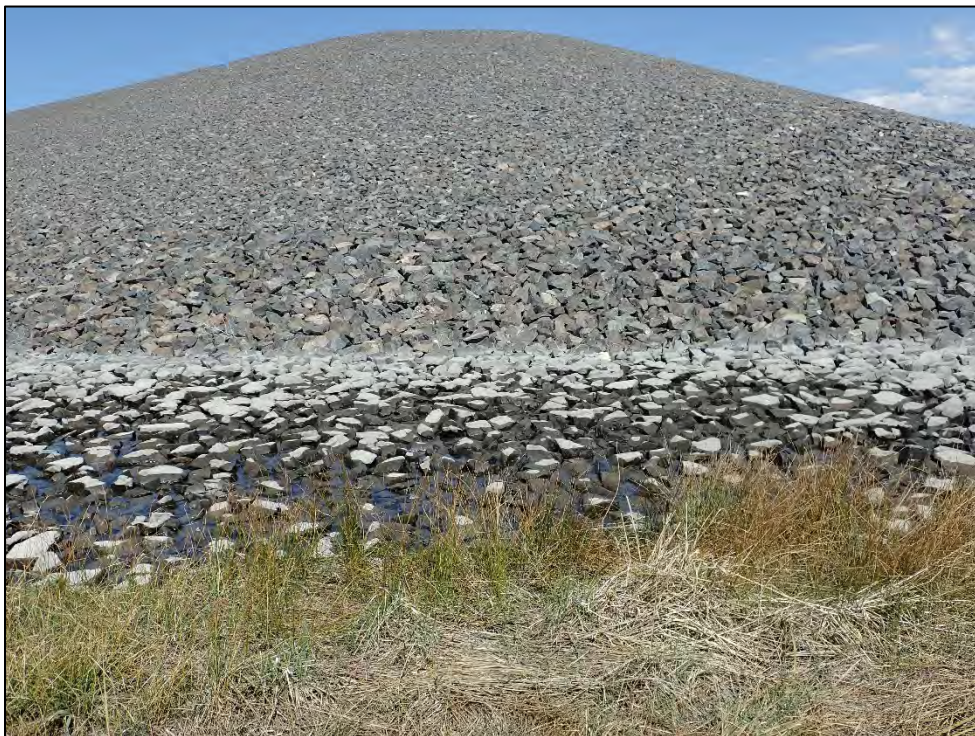
PL-6. Water in Cell Apron, Southeast Corner
