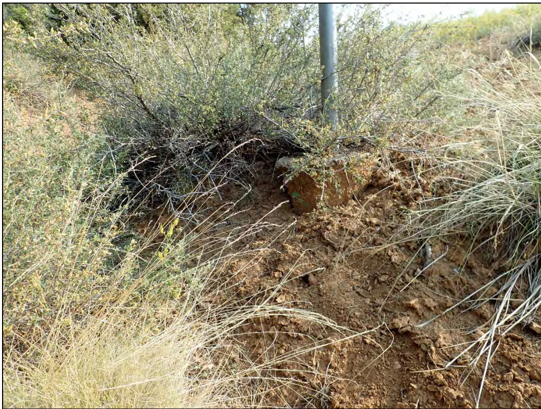
PL-2. Perimeter Sign P79 Undercut by Erosion
