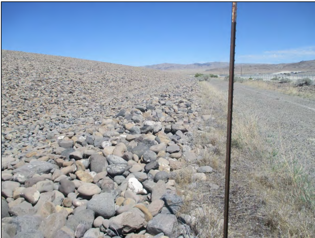
PL-4. Disposal Cell, South Side Toe Drainage
