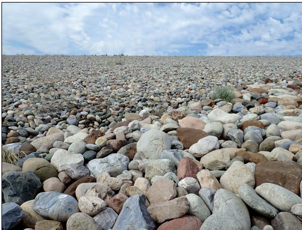
PL-8. Linear Depression in Cell Toe Slope
