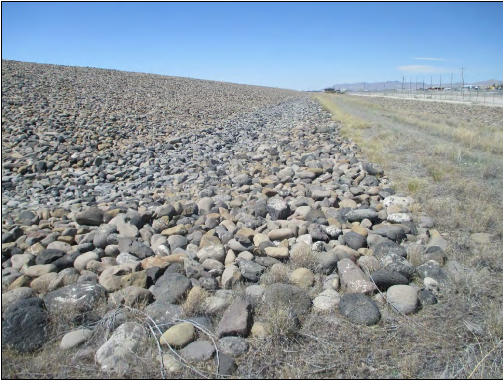
PL-5. Disposal Cell, East Side Toe Drainage
