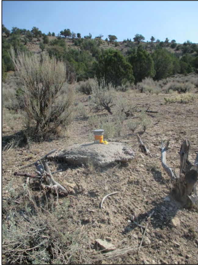
PL-3. Boundary Monument BM-18 with Undercutting
