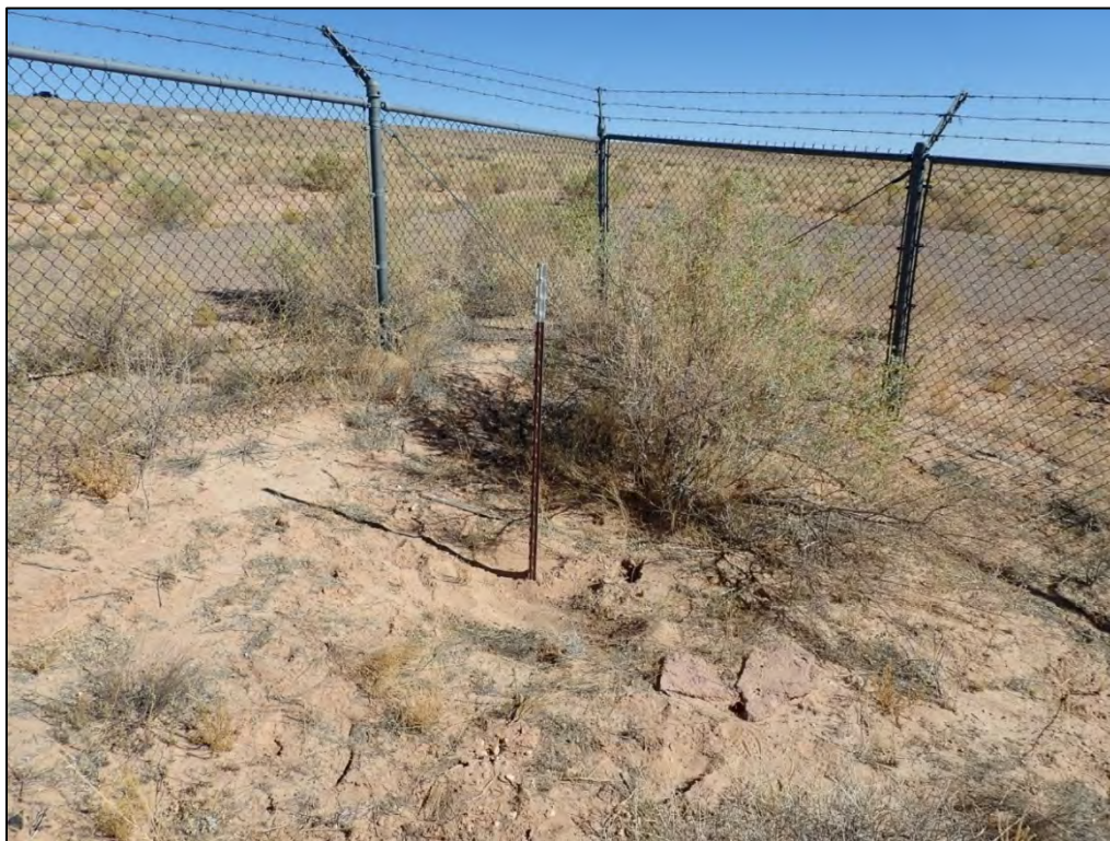
PL-6. Survey/Boundary Monument SM/BM-3 with Sand Accumulation
