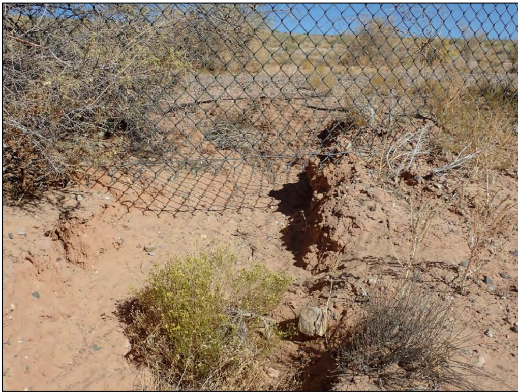
PL-3. Erosion Under Fence
