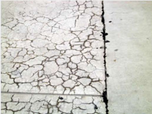
Alkali-silica reaction
