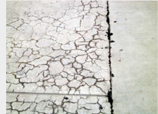
Alkali-silica reaction
