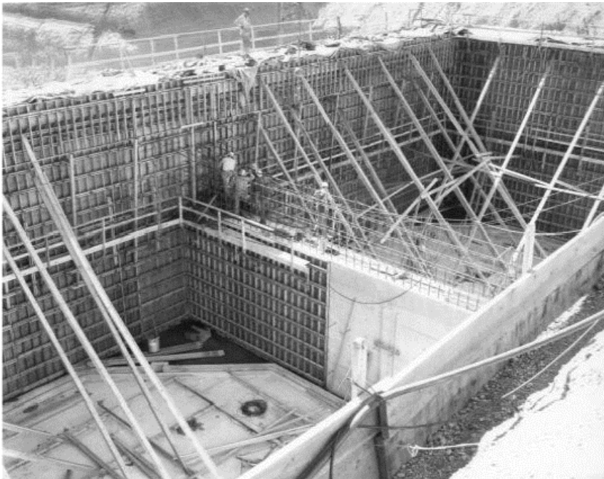
Figure 3-3. Monolithic square vault for Tank WM-190 (DOE, 2003)
