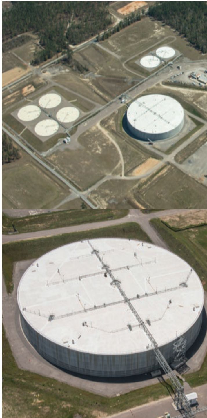
Figure 3-11. Saltstone disposal units: Closeup of the 121-million-L [32-million-gal] unit in the bottom image and all the units, including the smaller 11.4-million-L [3-million-gal] units in the top image (SRR, 2017)
