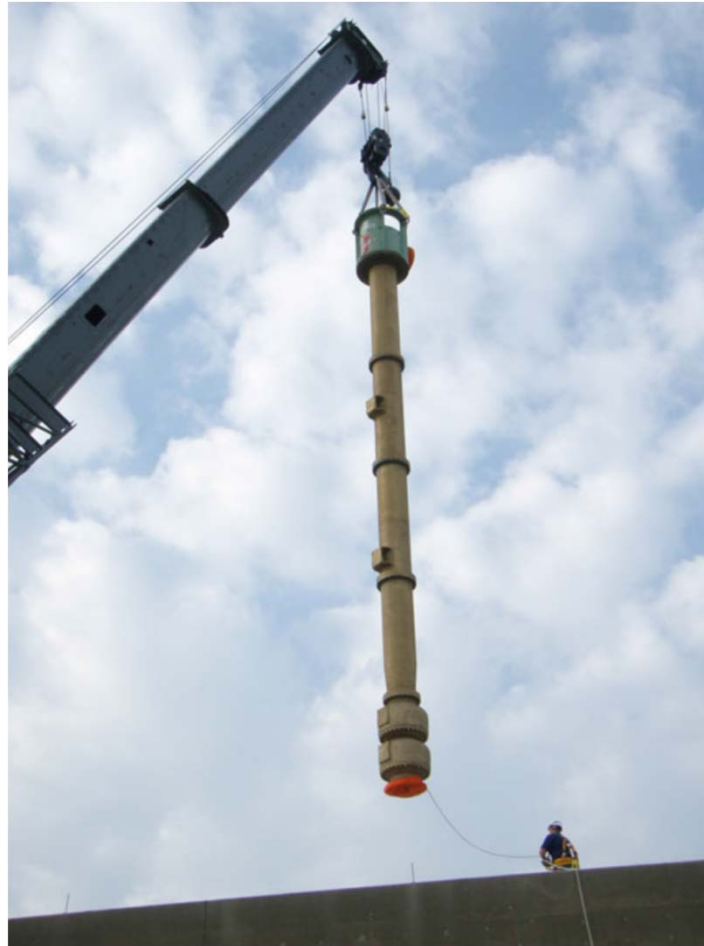
Figure 4 – SSW Pump 2-01 Replacement (April 2008)
