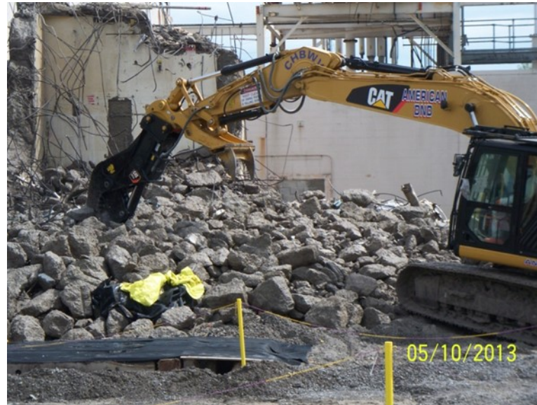
Processing and Size Reducing Concrete Rubble at 01-14
