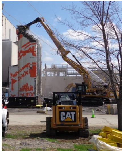
2 - 200,000 lb Class Excavator = Start of Demo at Top of Bldg (01-14 Demo)
