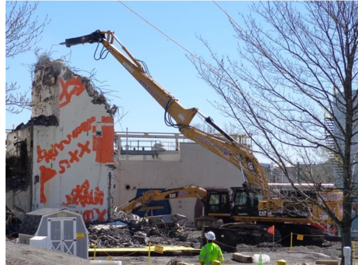
3 - 200,000 lb Class Excavator with Hydraulic Hammer (01-14 Demo)
