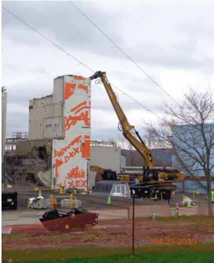
1 - Demo with 200,000 lb Class Excavator with Shear (01-14 Demo)
