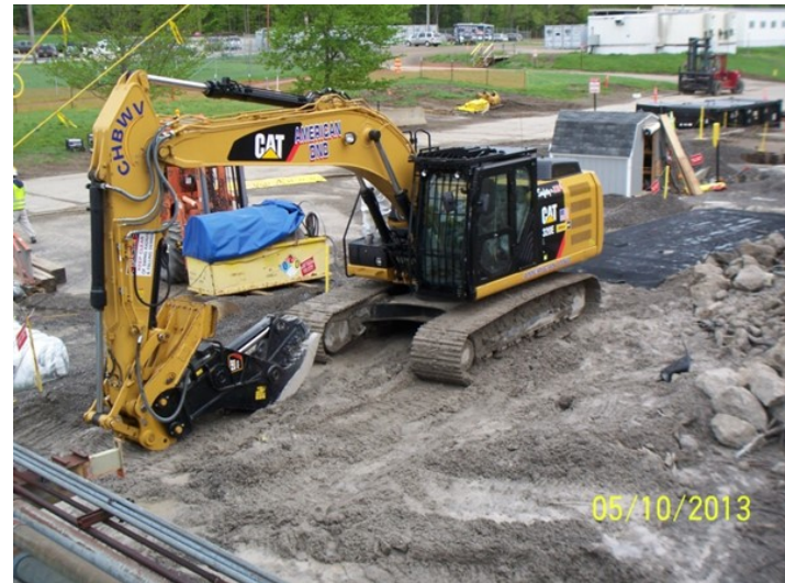
4 - 40,000 lb Class Excavator with Concrete Pulverizer
