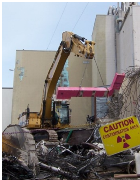
Selective Dismantling of Rad-component DURING 01-14 Demo
