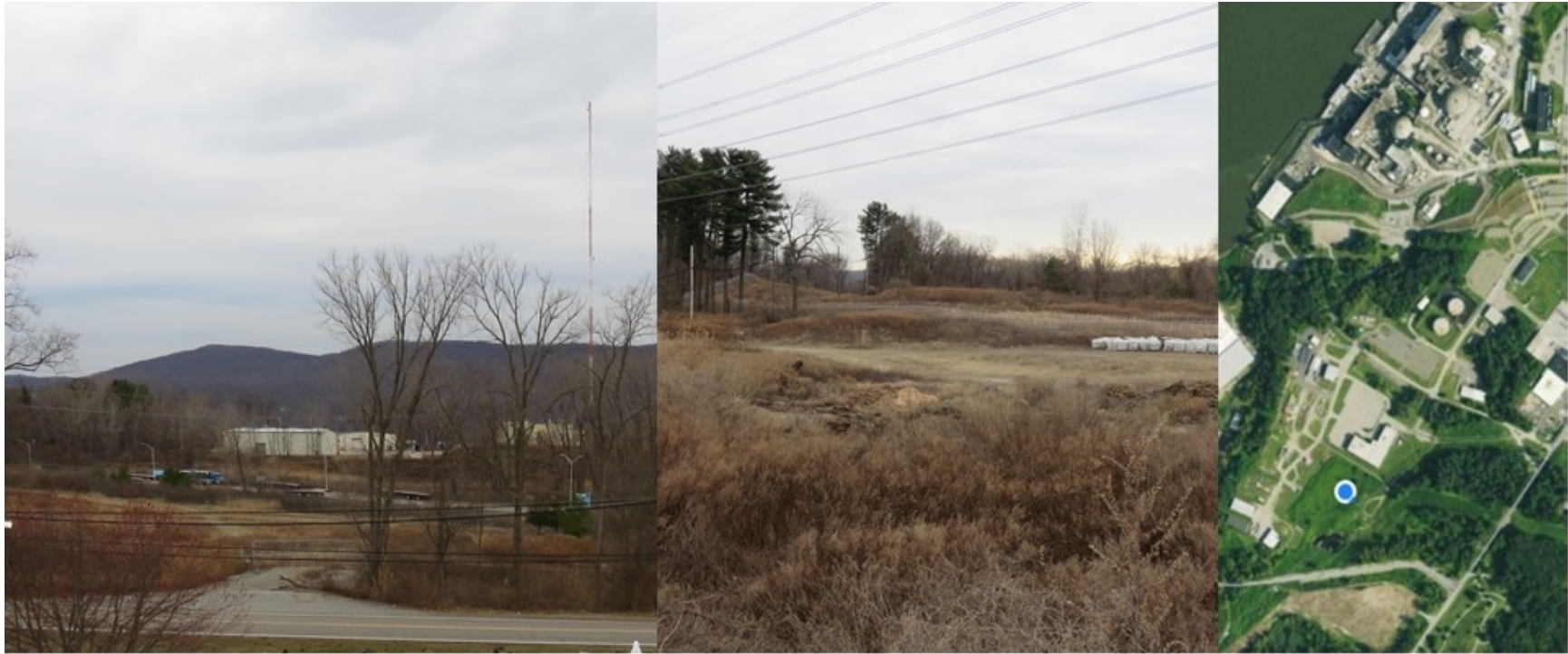
Figure 5. View of the 42-inch AIM pipeline from near Indian Point. At left is a view of the right of way from a location southeast of Indian Point. The pipeline area can be identified by the lighter grass beyond the trucks on the opposite side of the road (Broadway); the Indian Point SOCA is well outside the frame to the right; the red and white tower is the meteorology tower that Entergy assessed for pipeline rupture impacts. At center is a view of the right of way from within the Indian Point property. The pipeline area can be identified by the lighter grass beyond the fence (behind the white items); the Indian Point SOCA is well behind the viewer and to the left of the frame. The photos show the hilly terrain near the site, with the pipeline in a low area. The image at right shows the Indian Point site near the top, blue dot with the location where the center photo was taken, and cemetery in the clear area near the bottom right. The pipeline area can be identified by the clear-cut through the trees; the Buchanan switchyard is just to the right of the frame where the road (Broadway) intersects the edge of the image. The photos were taken by the team on March 12, 2020. (Right image: Imagery ©2020 Maxar Technologies, New York GIS, USDA Farm Service Agency, Map data ©2020 Google.)
