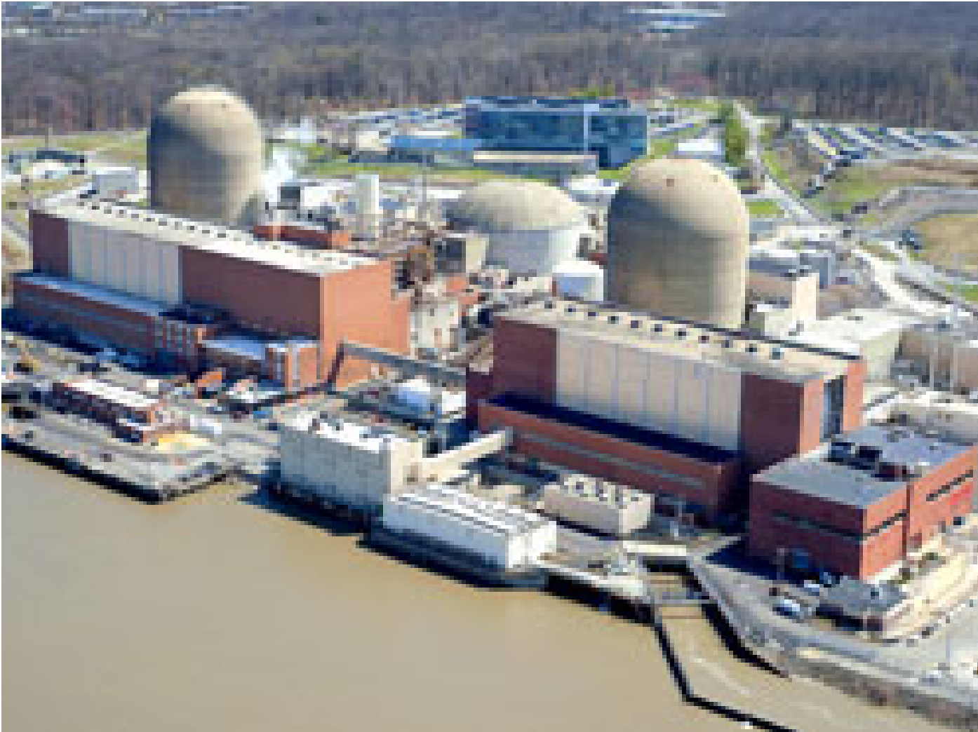
Figure 1. Aerial view of the Indian Point Energy Center on the east side of the Hudson River. This view shows the Unit 2 containment and turbine building on the left, the Unit 1 containment in the center, and the Unit 3 containment and turbine building on the right. (Some older aerial photos show a red and white stack associated with Unit 1; it has been removed and only the white base is showing to the left of Unit 1.)
