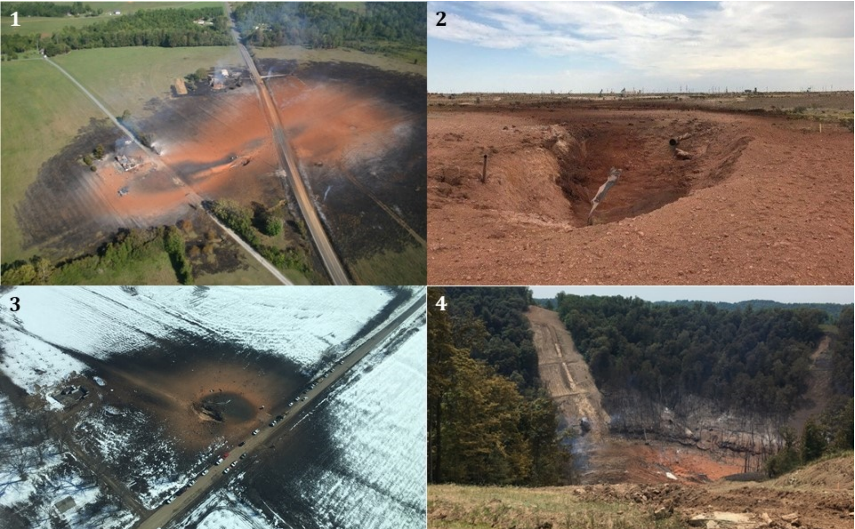
Figure 9. Pipeline rupture accident images obtained from PHMSA. Accident sites are: (1) Appomattox, VA in 2008, (2) Artesia, NM in 2019, (3) Mexico, MO in 2019, and (4) Moundville, OH in 2018.
