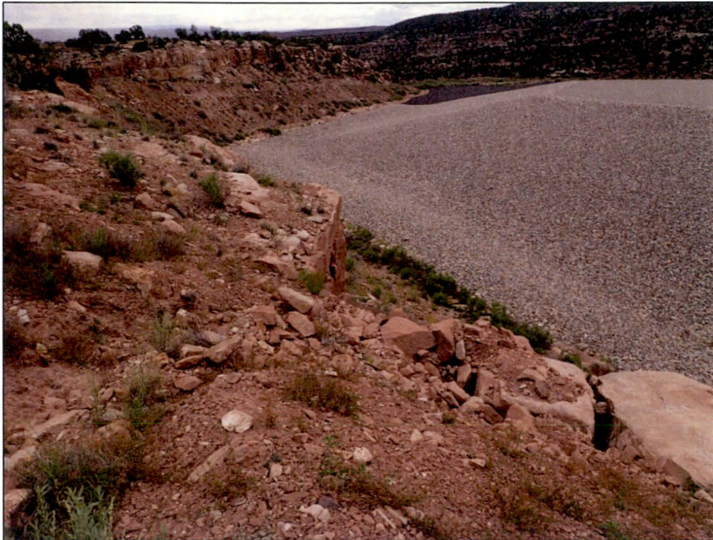
PL-11. Erosion Along Cliff Edge Above Disposal Cell
