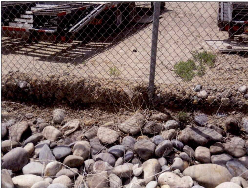
PL-2. Dirt Accumulation Against Perimeter Fence Between Perimeter Signs P11 and P12
