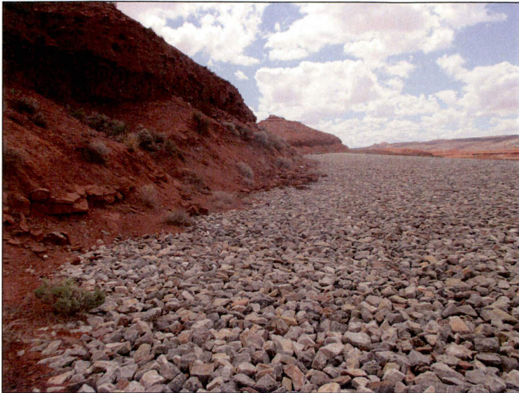
PL-5. Sloughed Rock on South Apron of Disposal Cell
