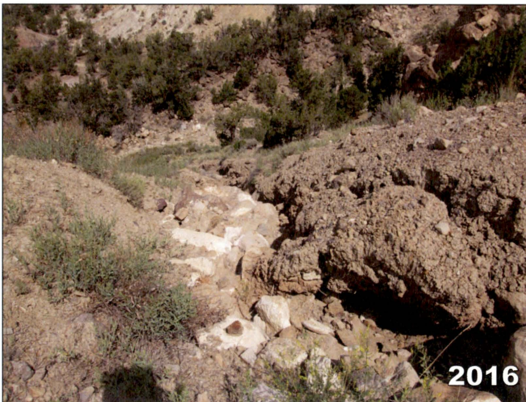
PL-10. (b) Erosion in Interceptor Trench Outfall Channel—2016 Photo for Comparison
