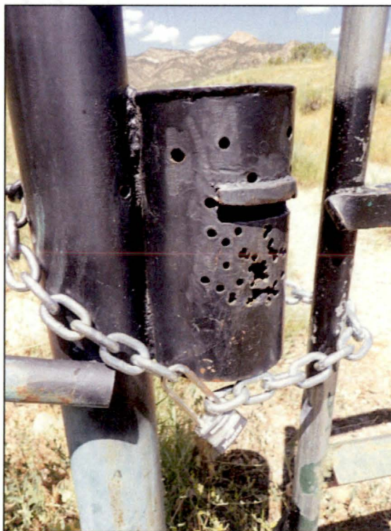
PL-2. Bullet Holes in Gate Cover at Outer Entrance Gate
