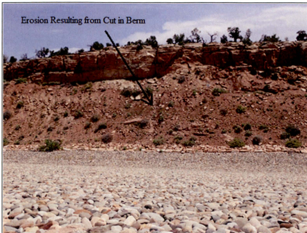
PL-13. Erosion Along Cliff from Cut in County Road EE22 Berm
