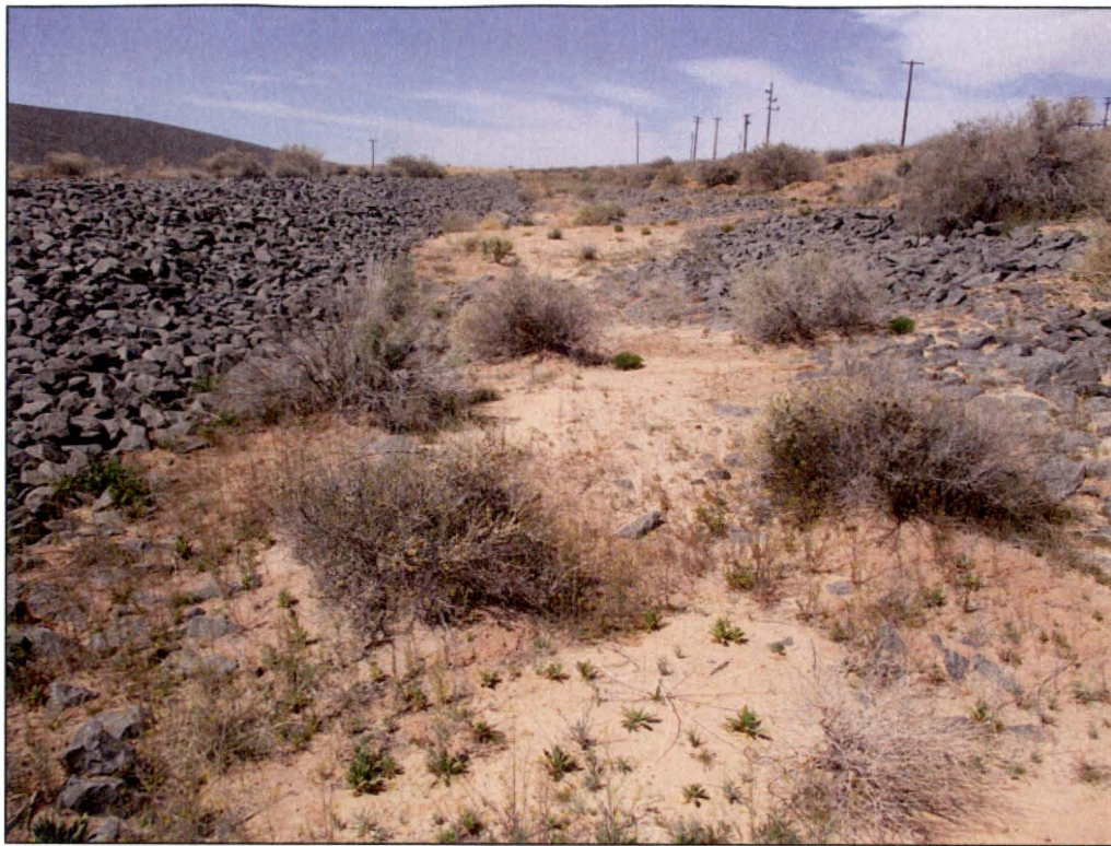
PL-15. Sediment Accumulation and Vegetation in Diversion Channel
