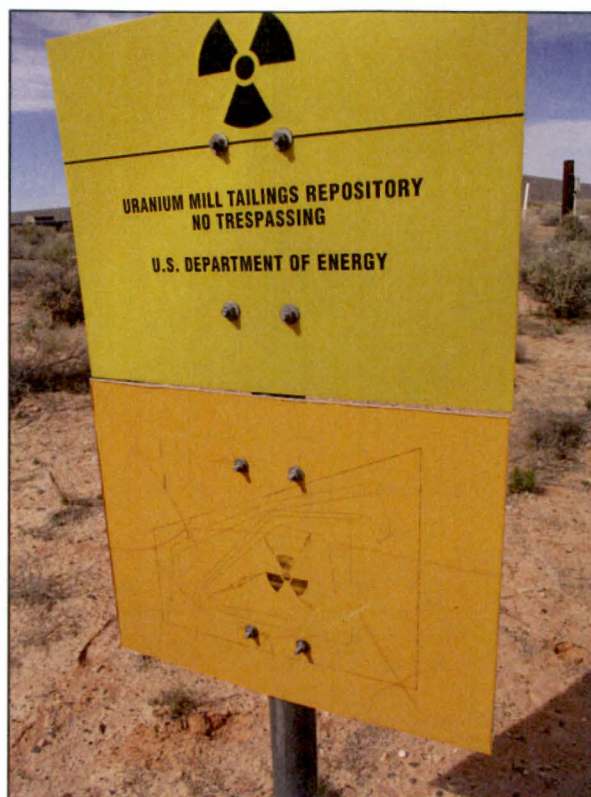
PL-9. Perimeter Sign P24; Pictorial Sign Faded (Replaced Following Inspection)
