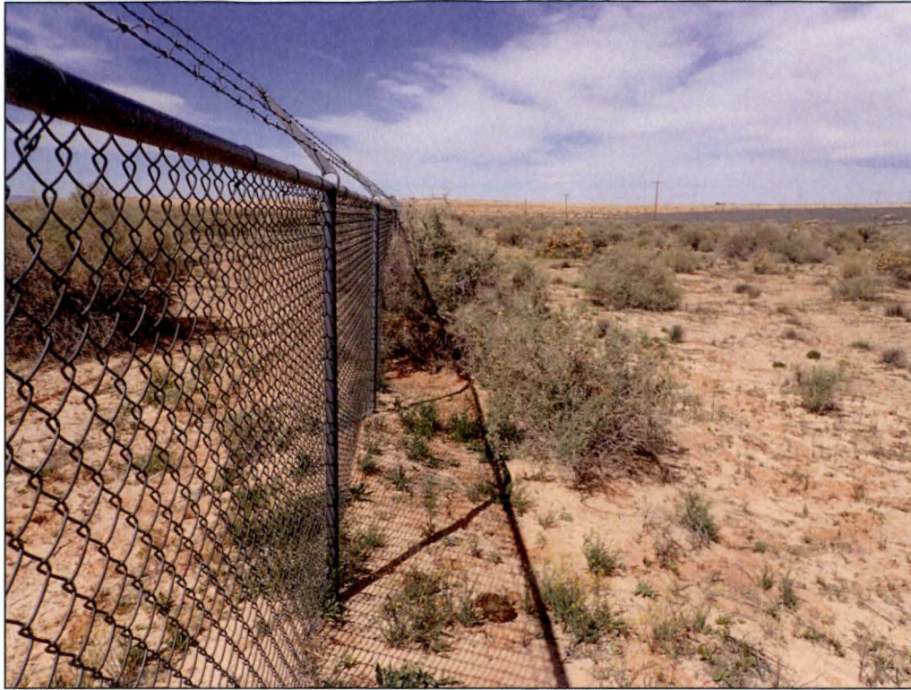
PL-7. Dense Shrub Growth on Perimeter Fence (Removed Following Inspection)
