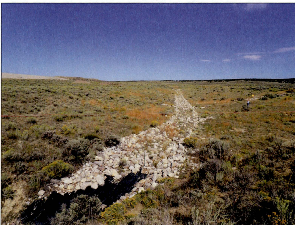
PL-10. Exposed Geotextile at Outlet to Swale No. 1
