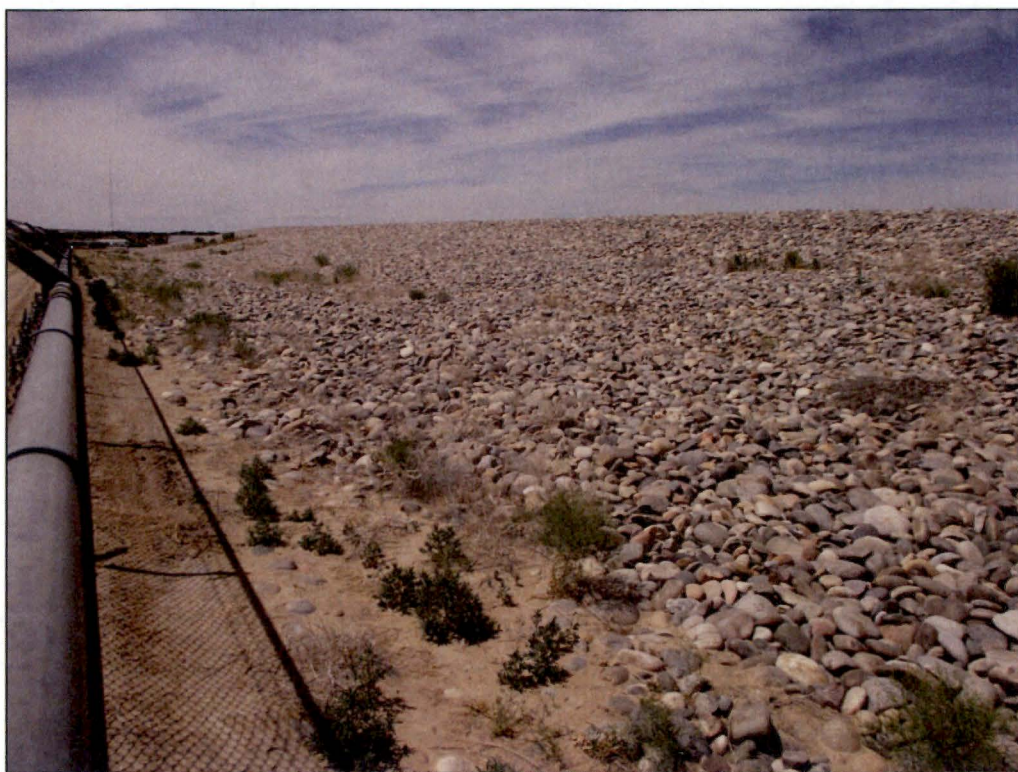
PL-7. Sediment Accumulation in Diversion Channel Along Southwest Slope of Disposal Cell
