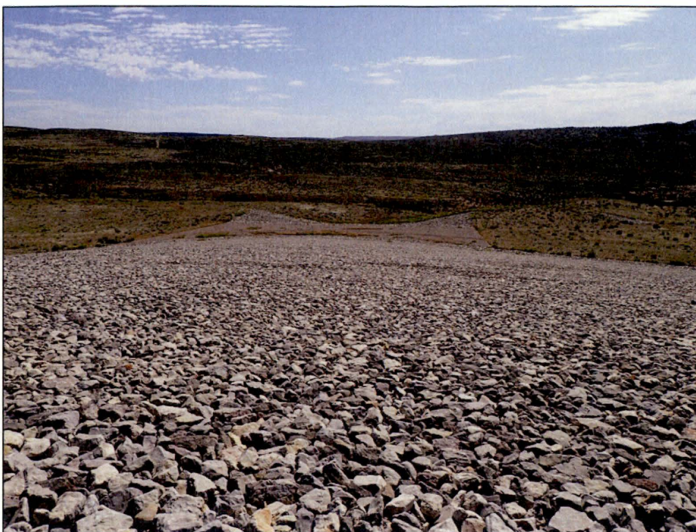
PL-9. Southeast Side Slope of Disposal Cell Side with Cobble Blanket in Background
