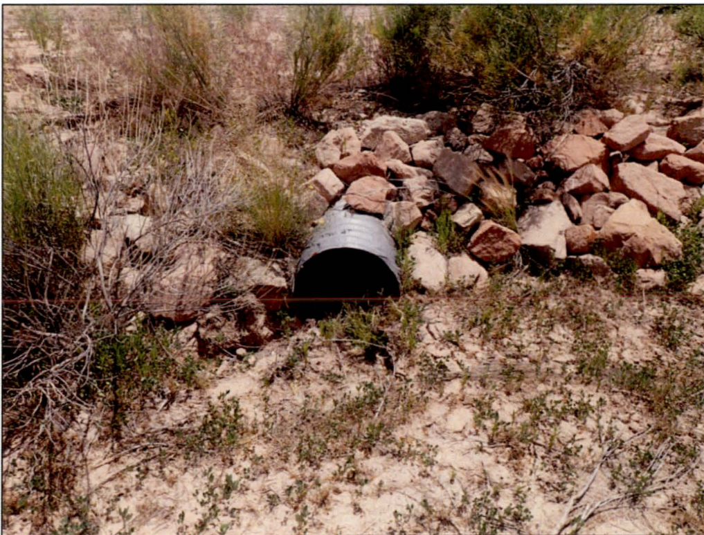
PL-10. Culvert Inlet Partially Blocked by Sediment
