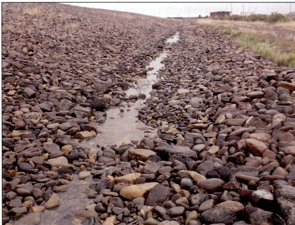
PL-15. Standing Water in Disposal Cell Toe Drainage
