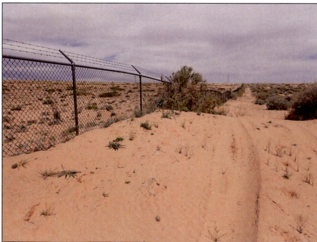
PL-4. Sand Accumulation Along Western Perimeter Fence and Road (Removed Following Inspection)
