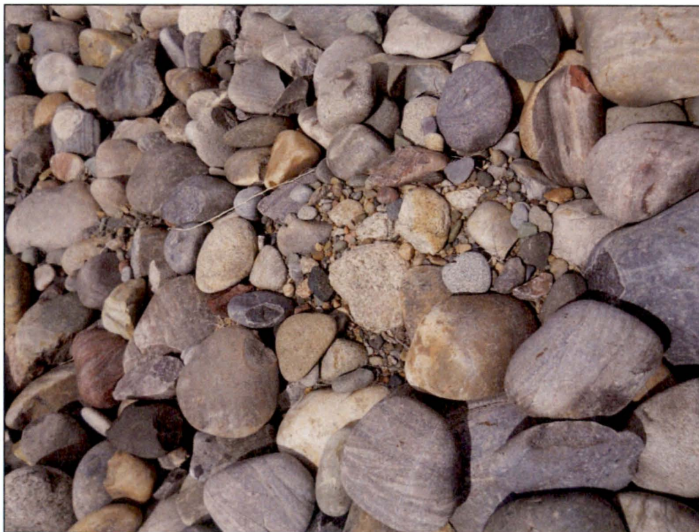
PL-6. Exposure of Smaller Cobbles and Gravels Along Ridge of Disposal Cell
