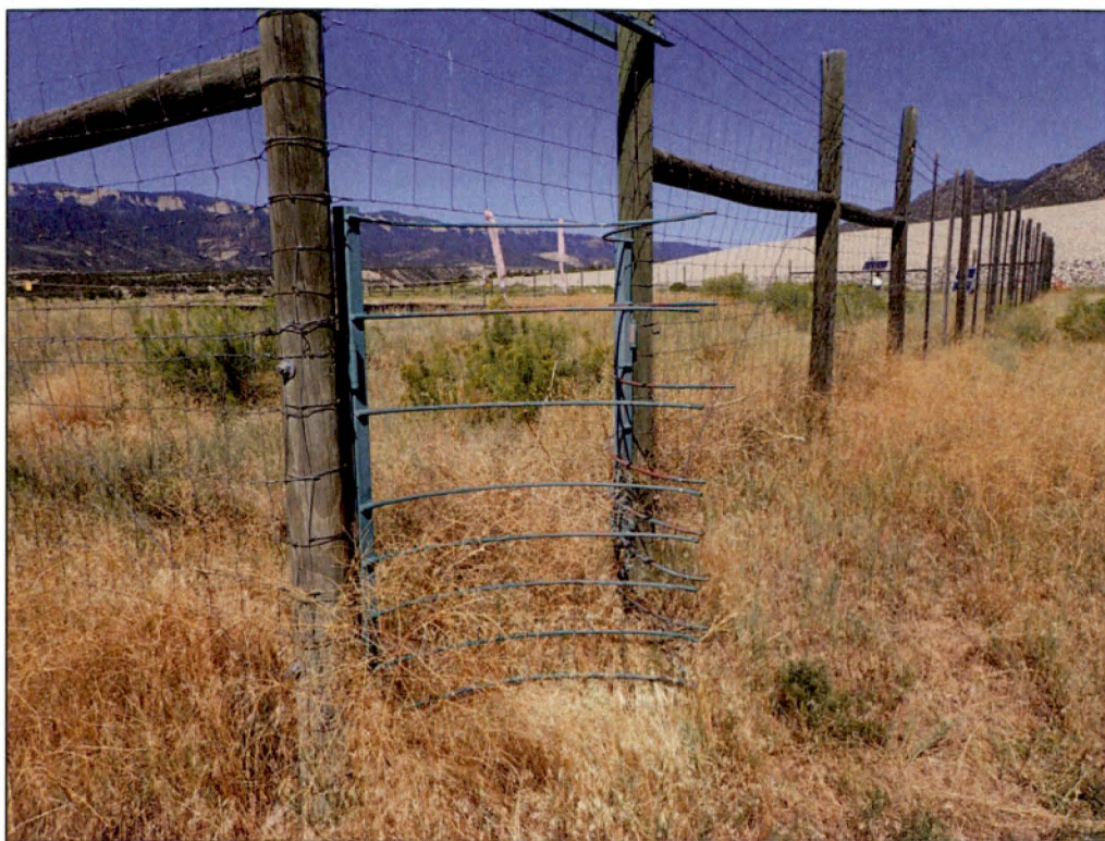
PL-5. Tumbleweed Buildup in Wildlife Gates (Removed Following Inspection)
