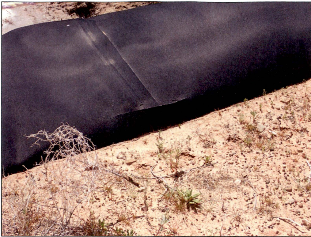
PL-19. Crack in Evaporation Pond Liner (Repaired)
