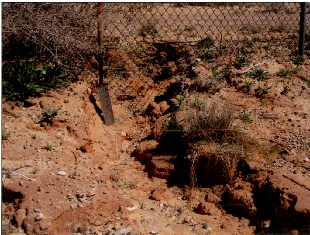
PL-6. Soil Erosion Under Perimeter Fence Between Perimeter Signs P27 and P28 (Repaired Following Inspection)
