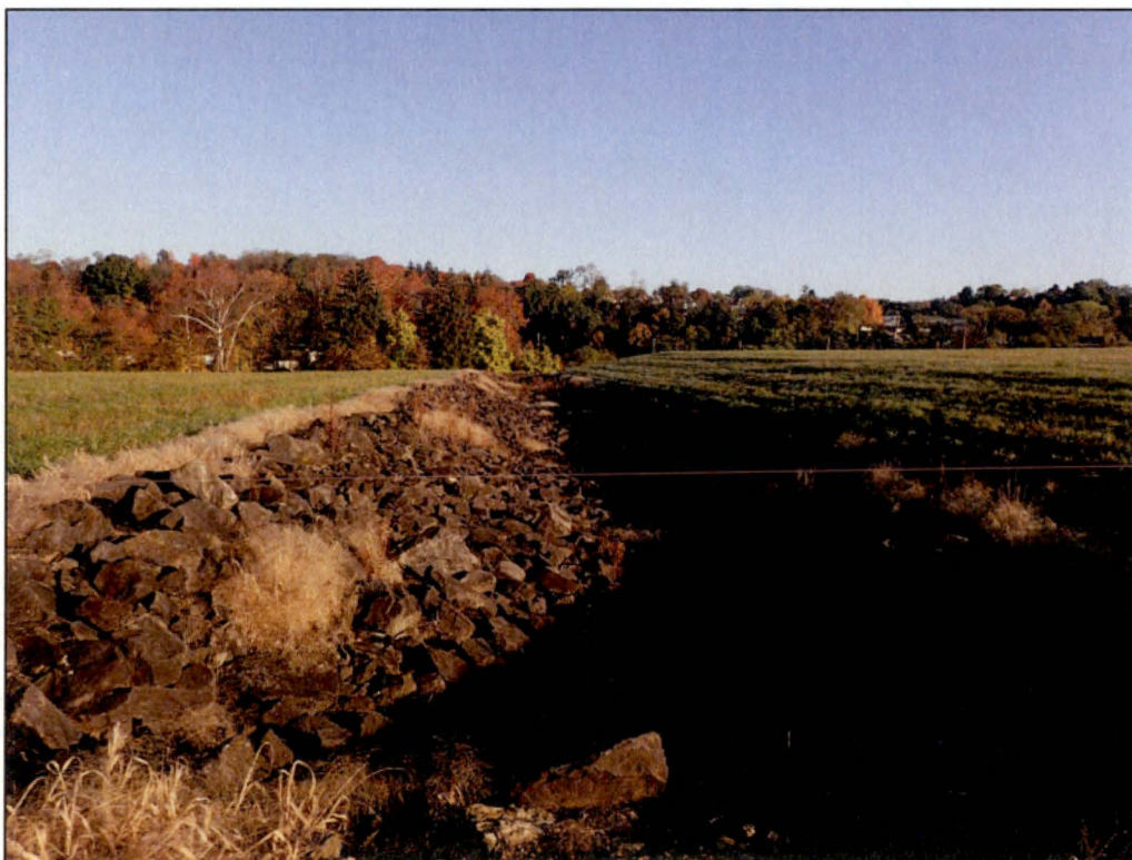
PL-4. West Section of Riprap-Armored Diversion Ditch
