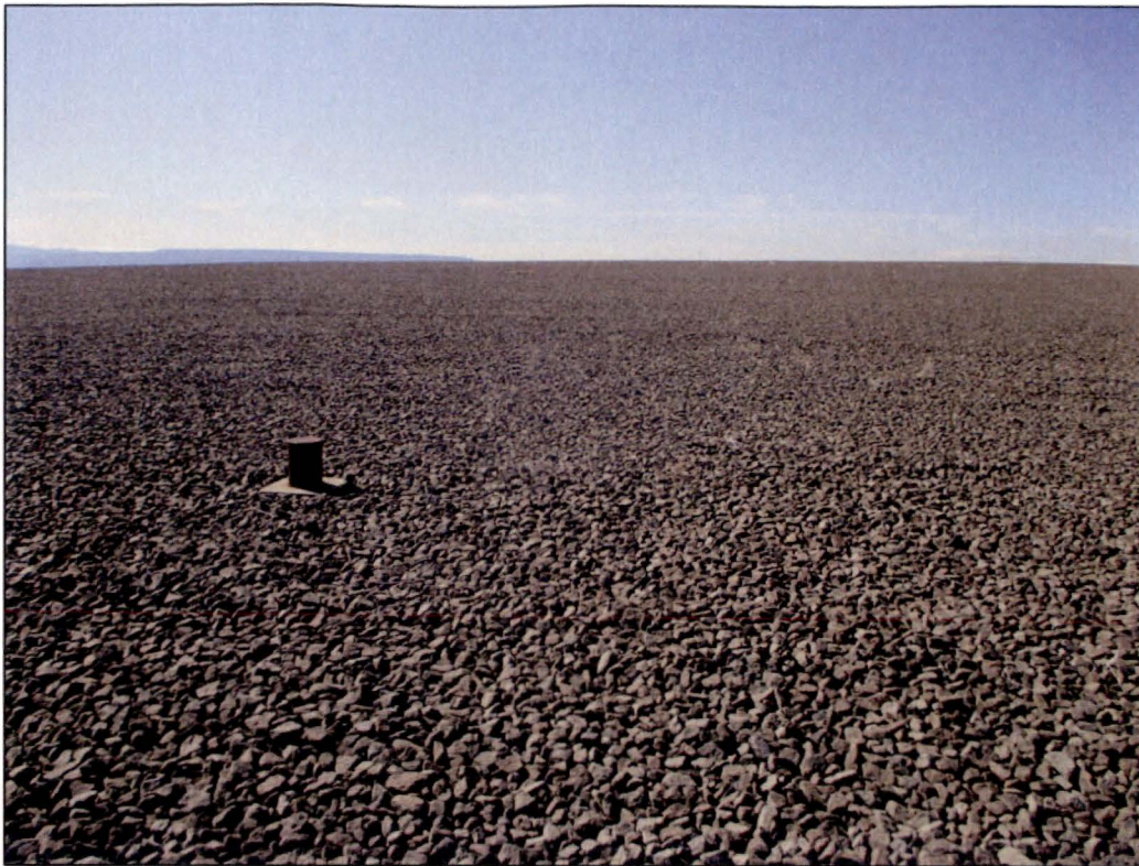
PL-7. Minor Settlement near Settlement Plate SP-4
