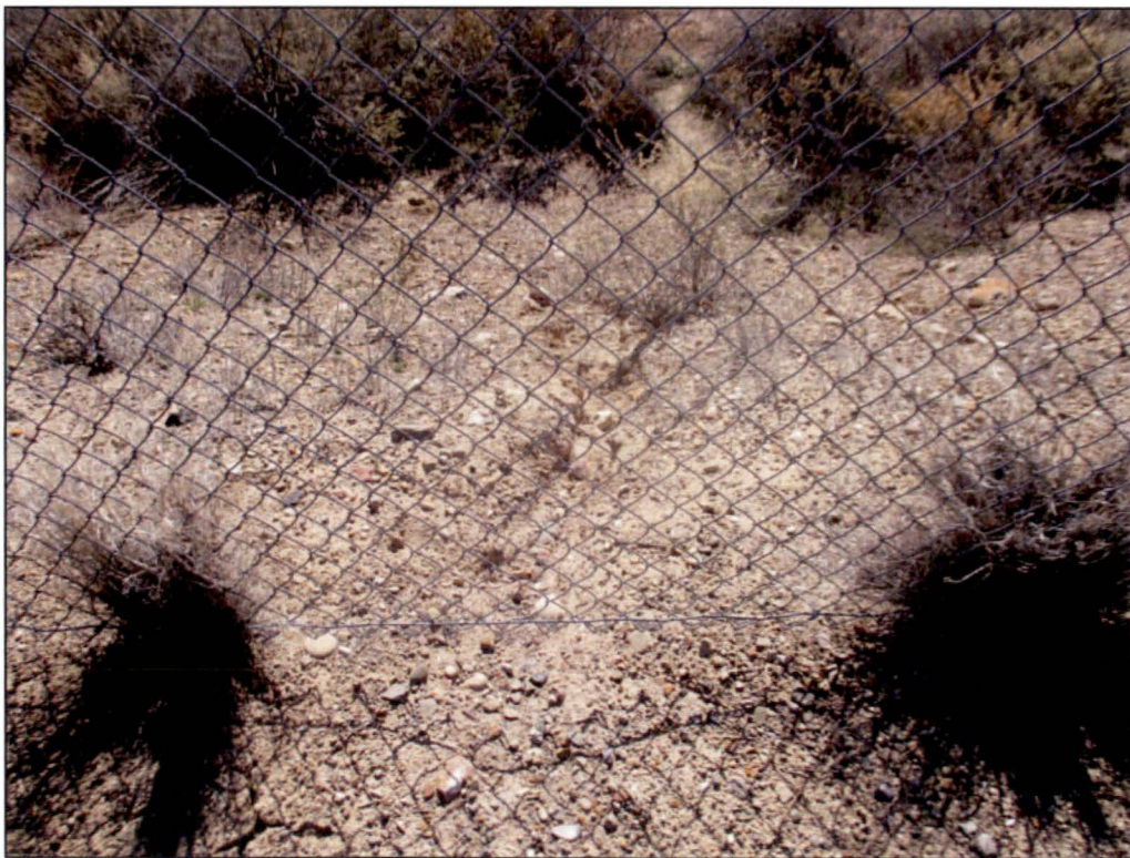
PL-2. Minor Erosion Under Southeast Security Fence Line (Repaired)
