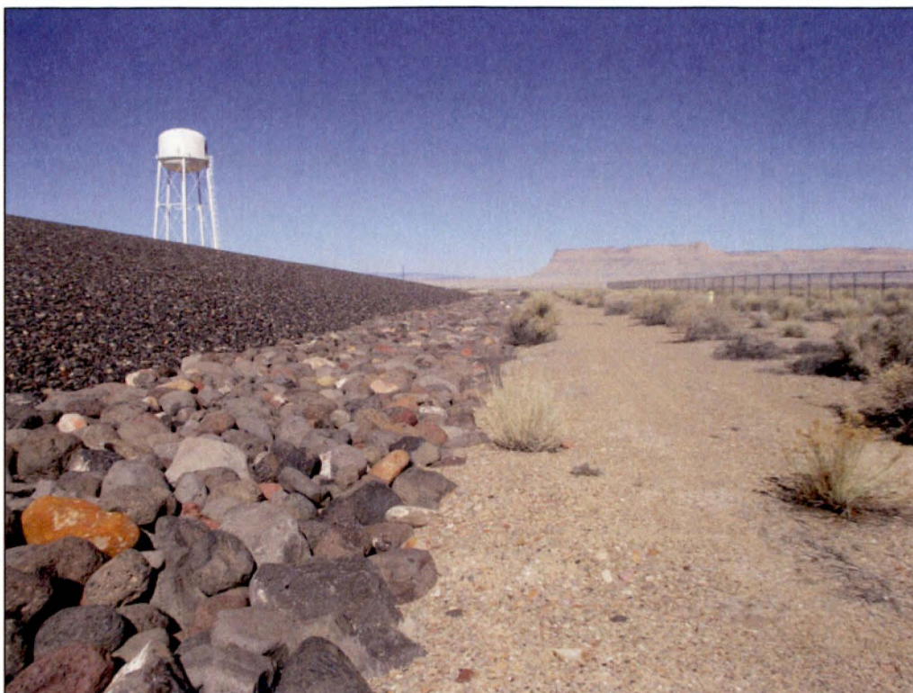
PL-7. Apron Along Northeast Side of Disposal Cell
