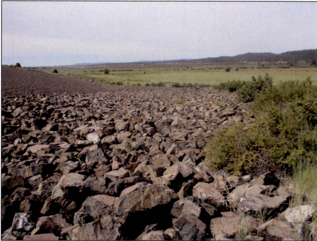
PL-11. Energy Dissipation Area Downstream of Drainage Channel North of Disposal Cell
