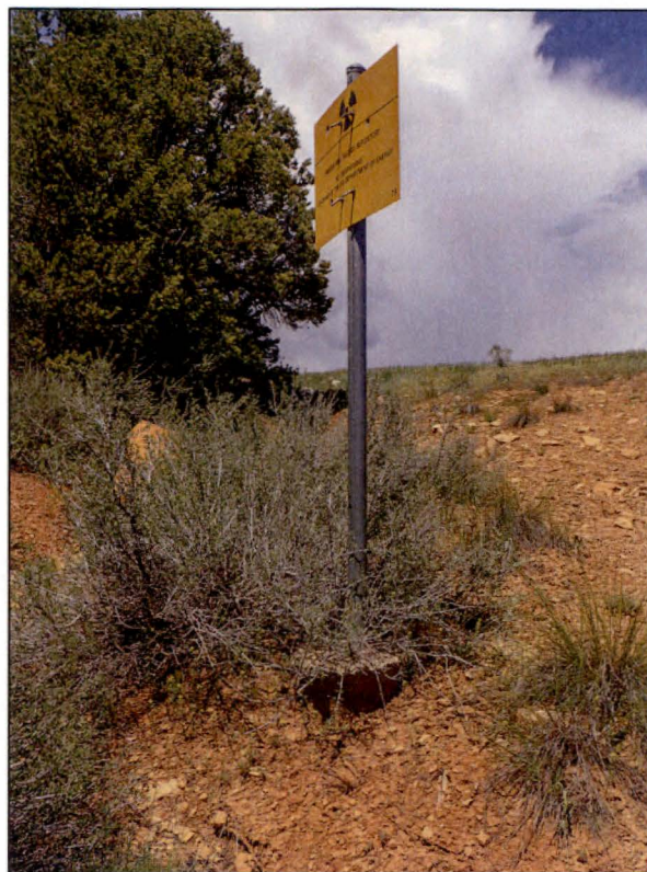
PL-1. Concrete Base of Perimeter Sign P79 (Undercut by Erosion)
