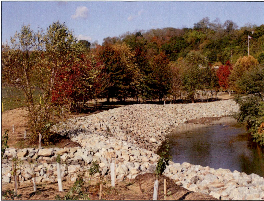
PL-5. Newly Repaired Riprap Embankment
