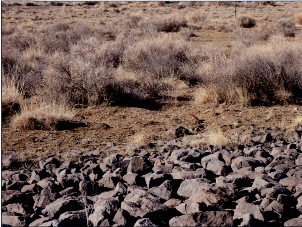
PL-9. Rills at Southern Base of Disposal Cell
