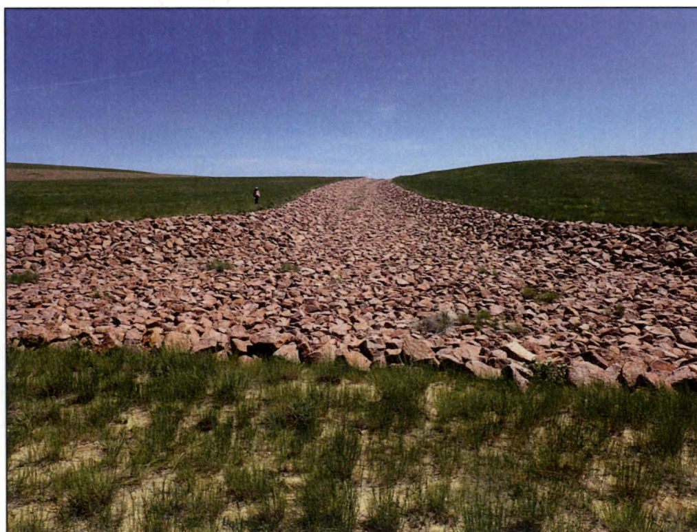
PL-12. Riprap-Armored Diversion Channel
