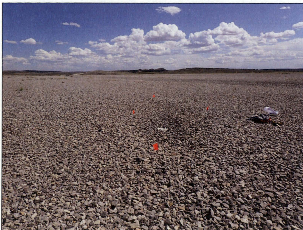
PL-6. Depression Feature on Top of Disposal Cell
