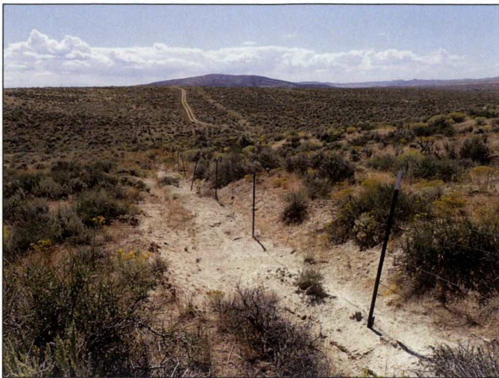
PL-1. Erosion Along Southwest Perimeter Fence
