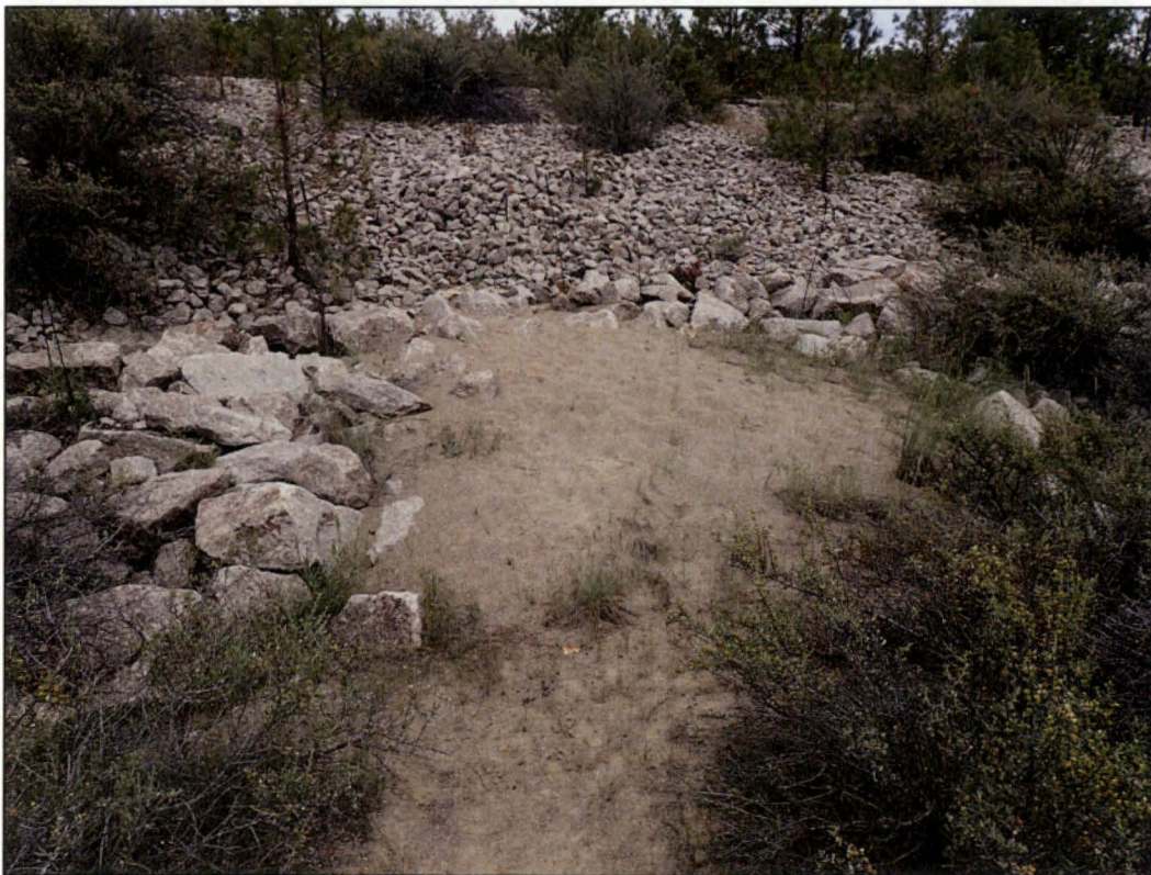
PL-8. Sand Deposit at Toe of Containment Dam Outslope
