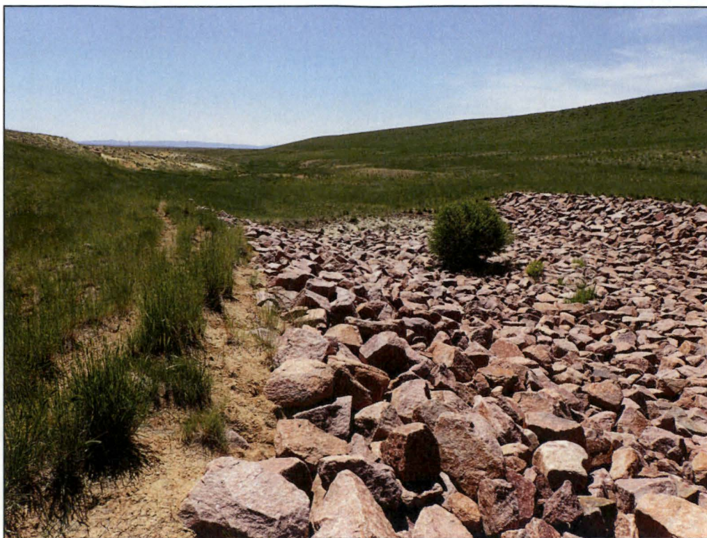
PL-13. Outlet of Riprap-Armored Diversion Channel
