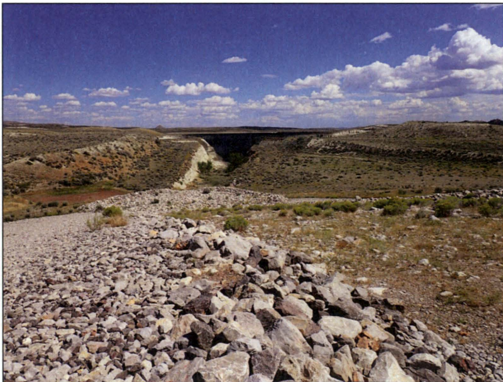
PL-16. Launch Rock Erosion Protection Basin on Disposal Cell East Side Slope; Rob Pit in Background
