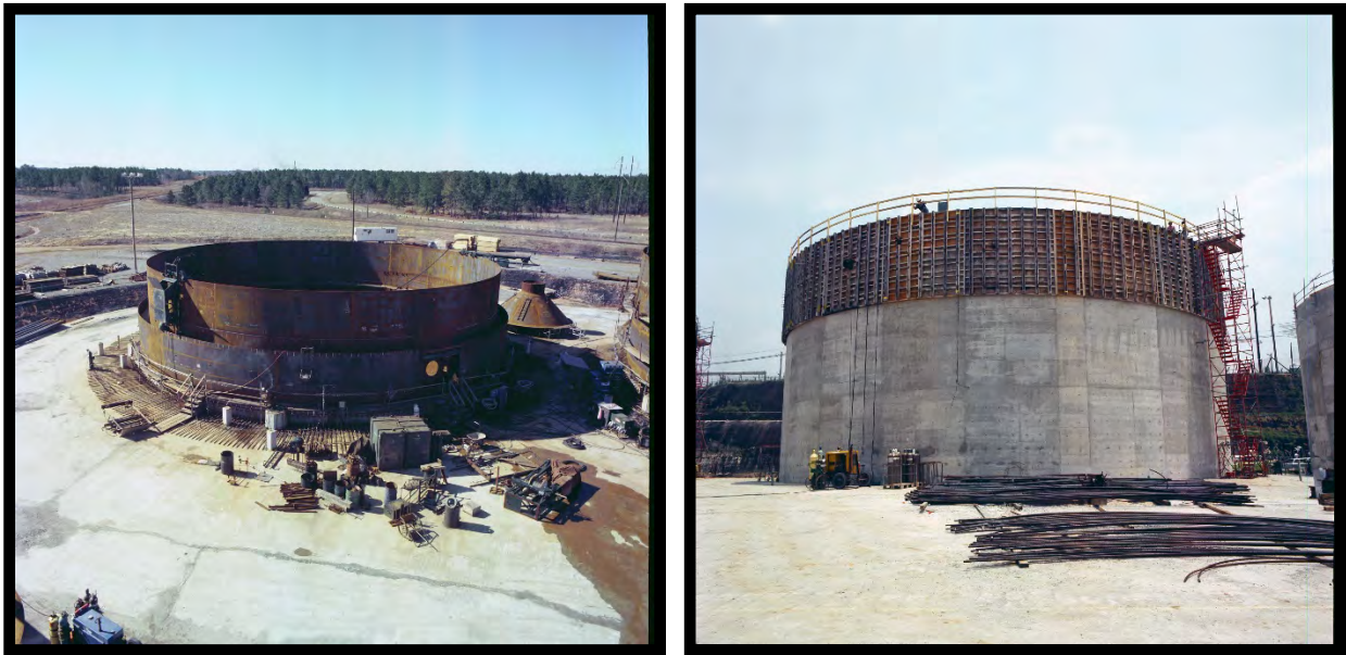
Figure 3.4-1: Typical Construction of Type III/IIIA Tanks
