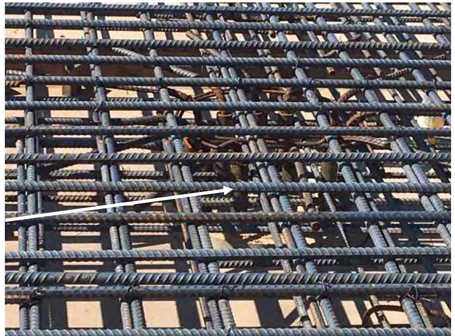
Roof - Column Reinforcing Bar Tie-In (Typical)
