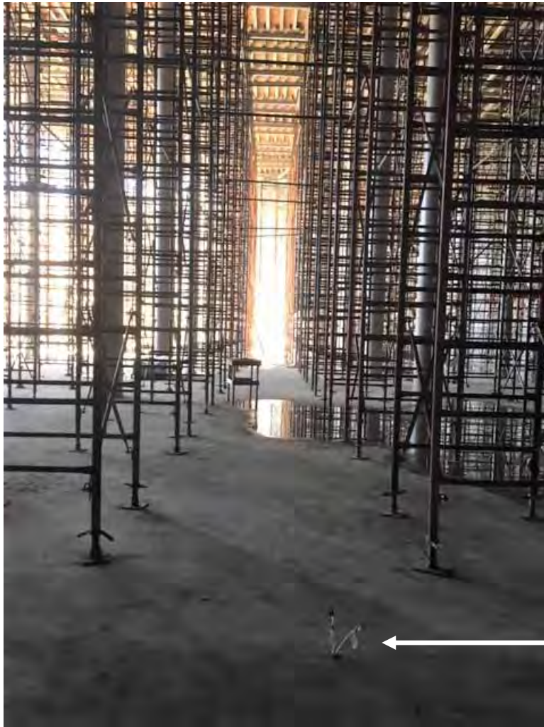
SDU 7 Interior Looking East
