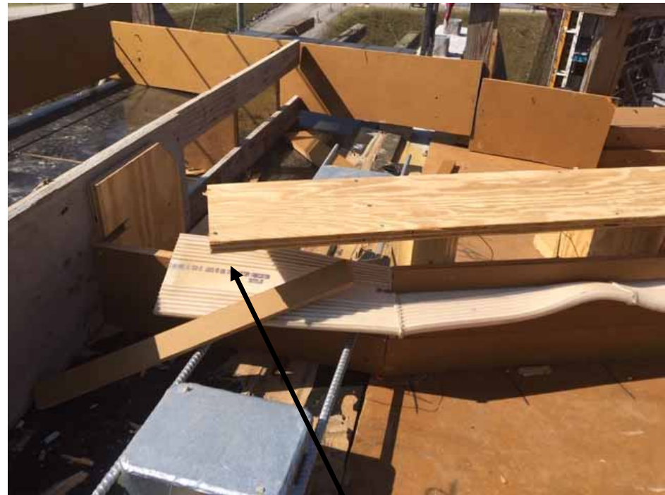
Water Stop at Edge of Roof
