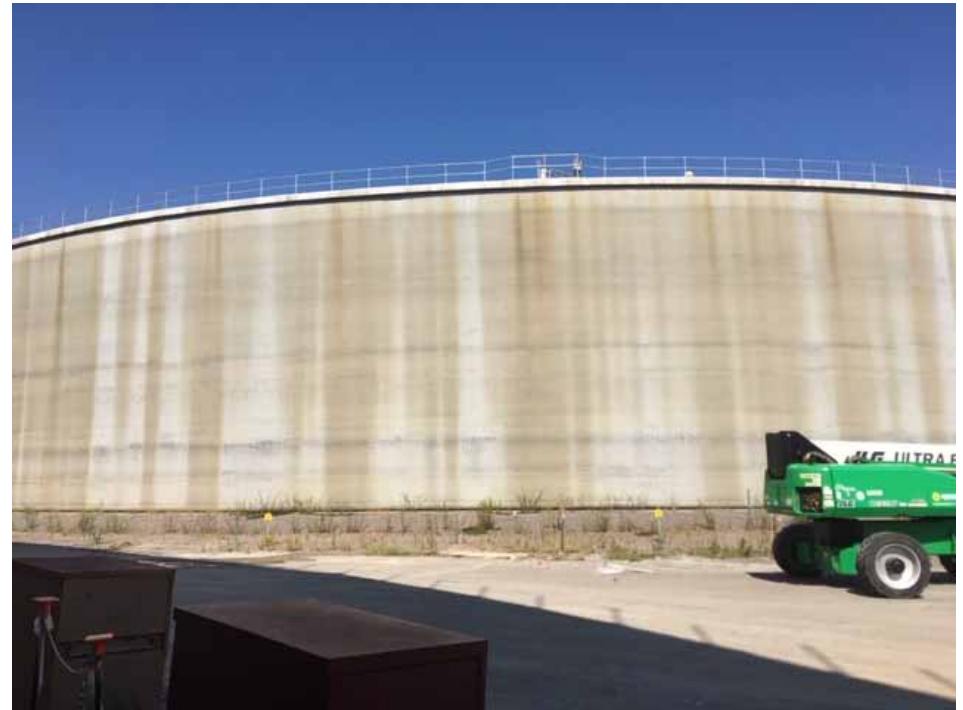
Looking North from SDU 7 Ground Level
