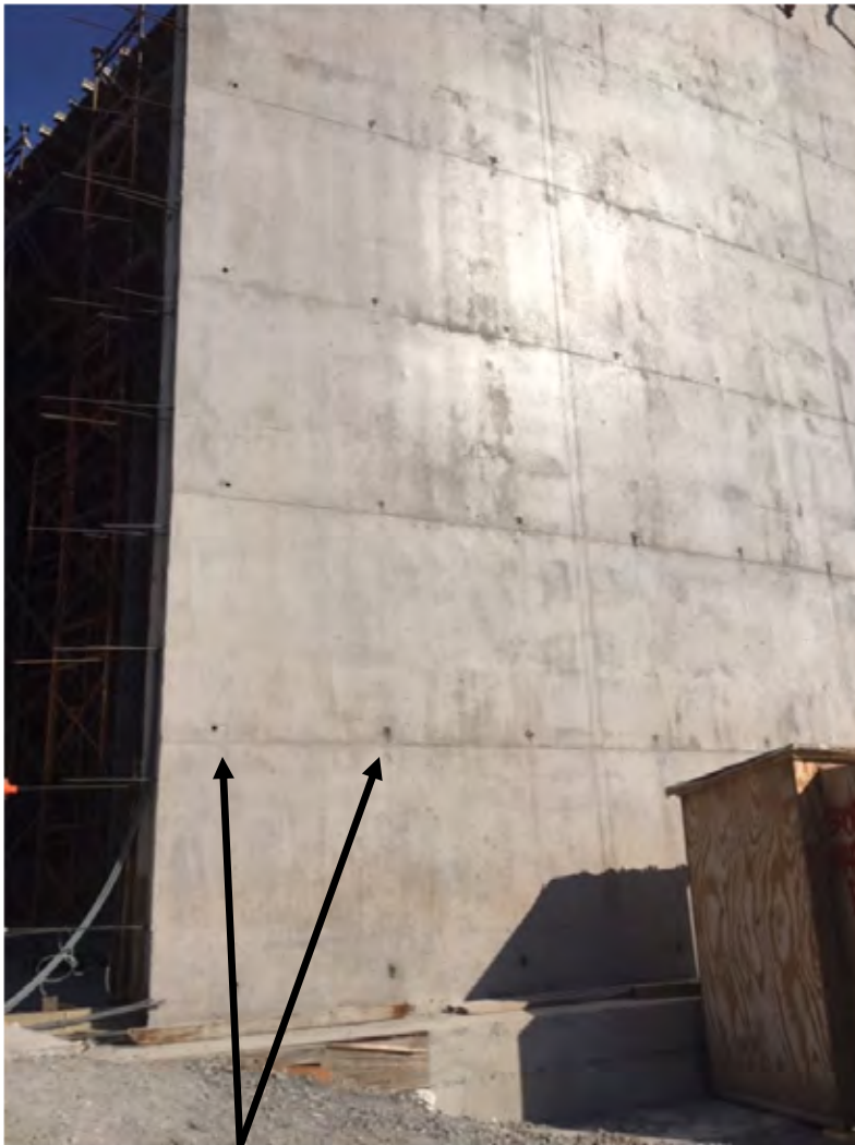
Form Tie Holes
