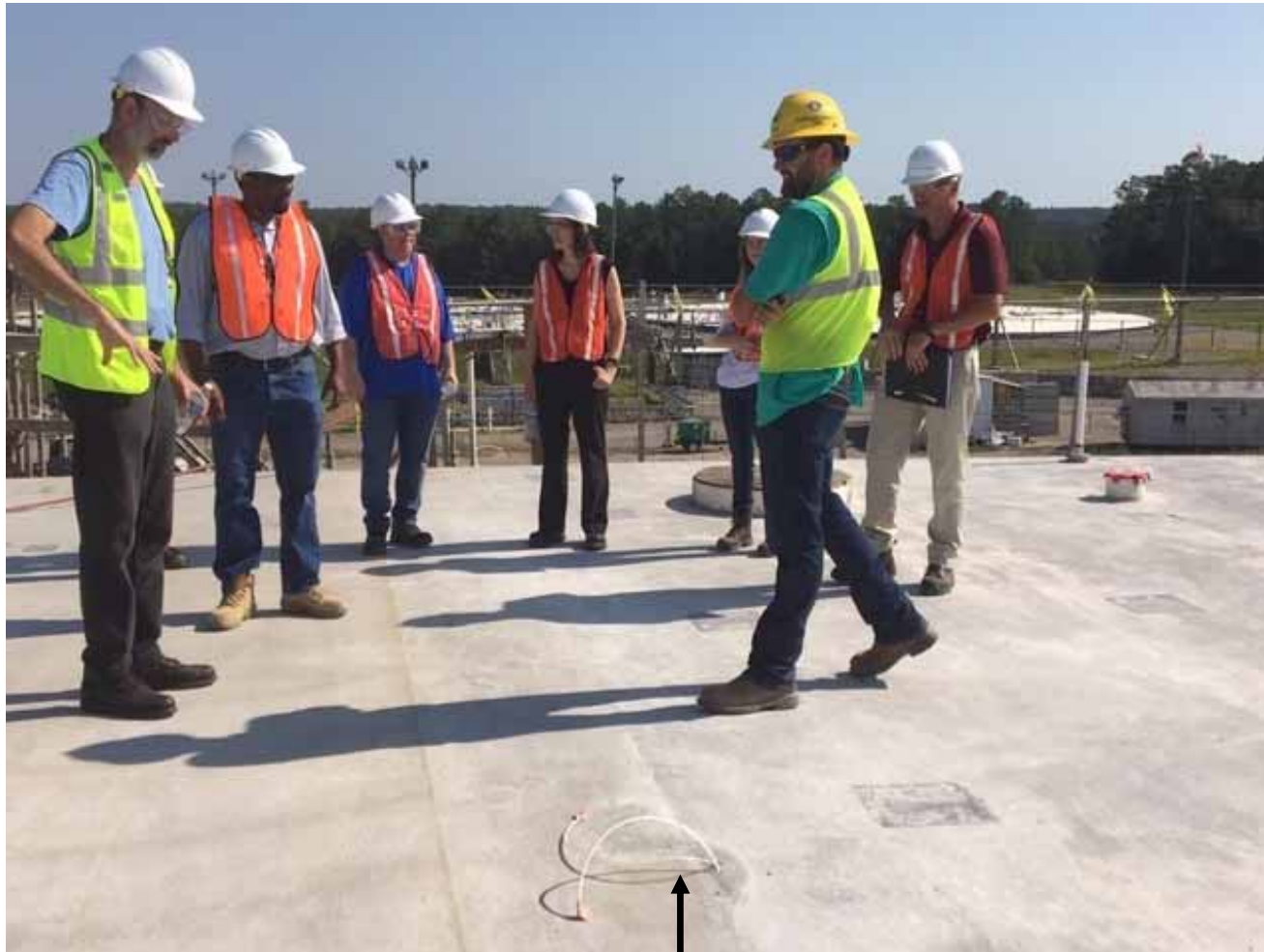
Epoxy Injection Tubing - Roof
