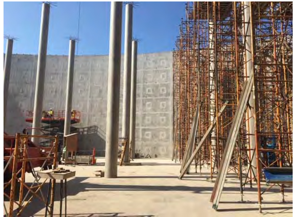
SDU 7 Interior Looking East
