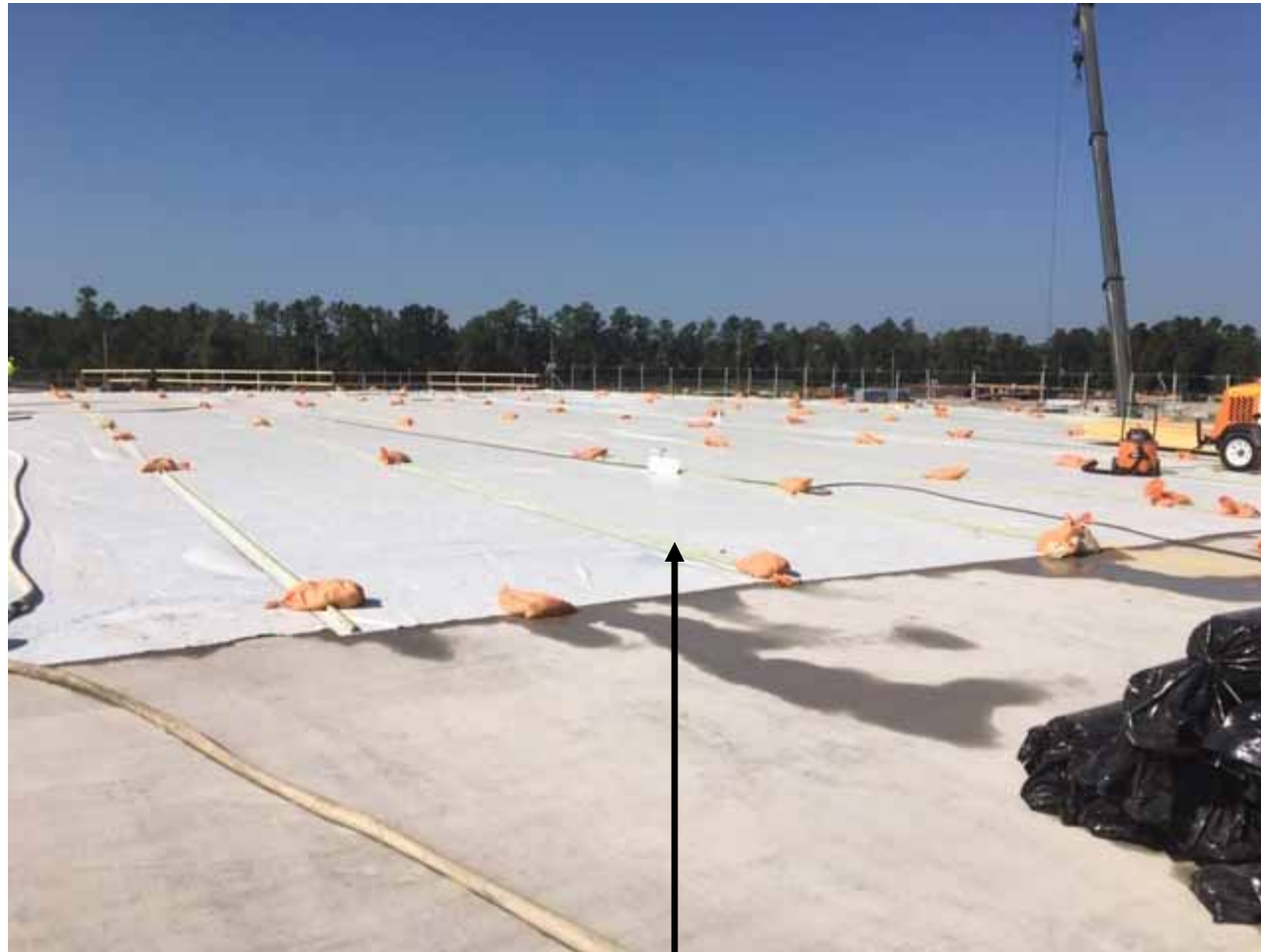
Roof Section #3 Under Water Cure
