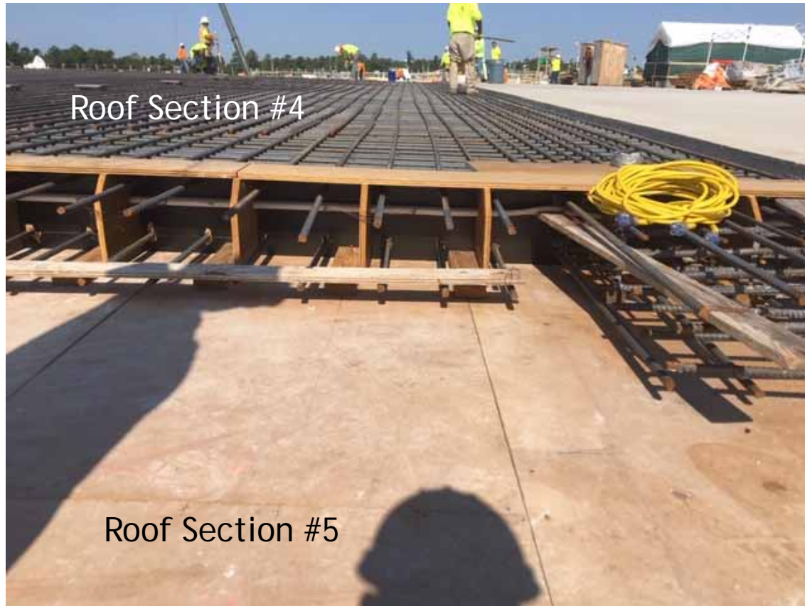
Roof Section #4 Reinforcing Bar Installation
