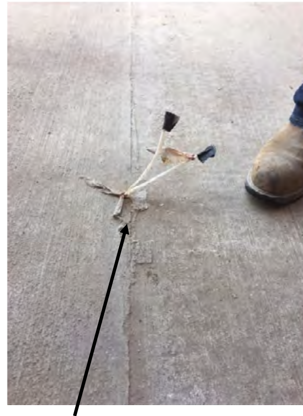
Epoxy Injection Tubing - Floor
