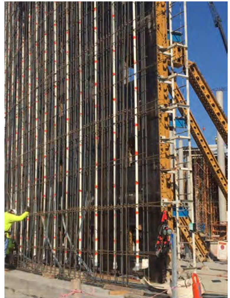
Wall Form Bracing
