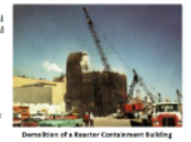
Demolition of a Reactor Containment Building
