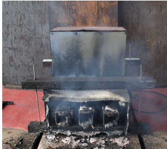
Bus Duct Testing 2016
