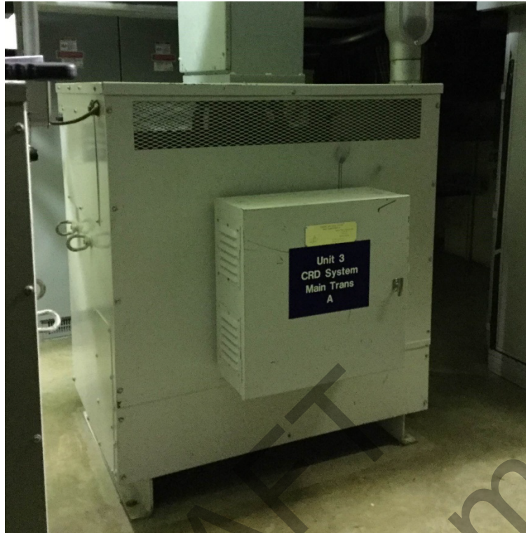
Figure 5-15 Example of Typical Dry-Type Transformer, Mid Range (375 kVA)
