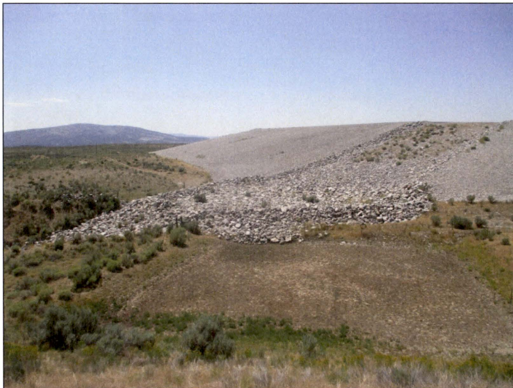
PL-14. Diversion Channel No. 1 Outlet and East Side Slope; Launch Rock Erosion Protection Basin
