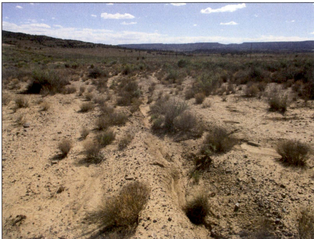
PL-17. Erosion East of Riprap Cutoff Wall at Outlet of North Channel
