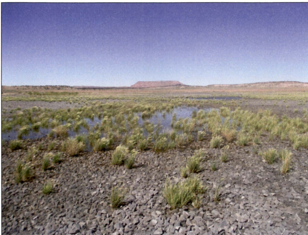
PL-7. Ponded Water on Main Tailings Disposal Cell Top Slope
