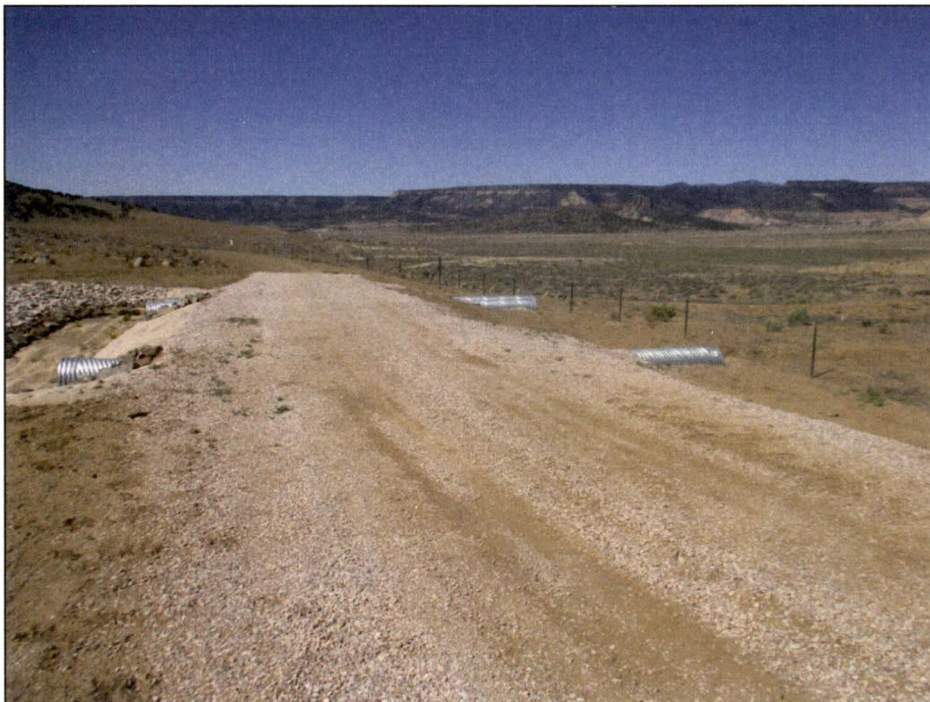
PL-22. Culverts Constructed in 2016
