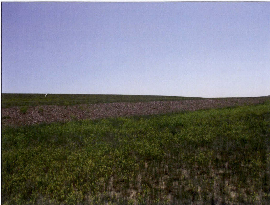
PL-9. Riprap-Armored Dam Outslope of Disposal Cell
