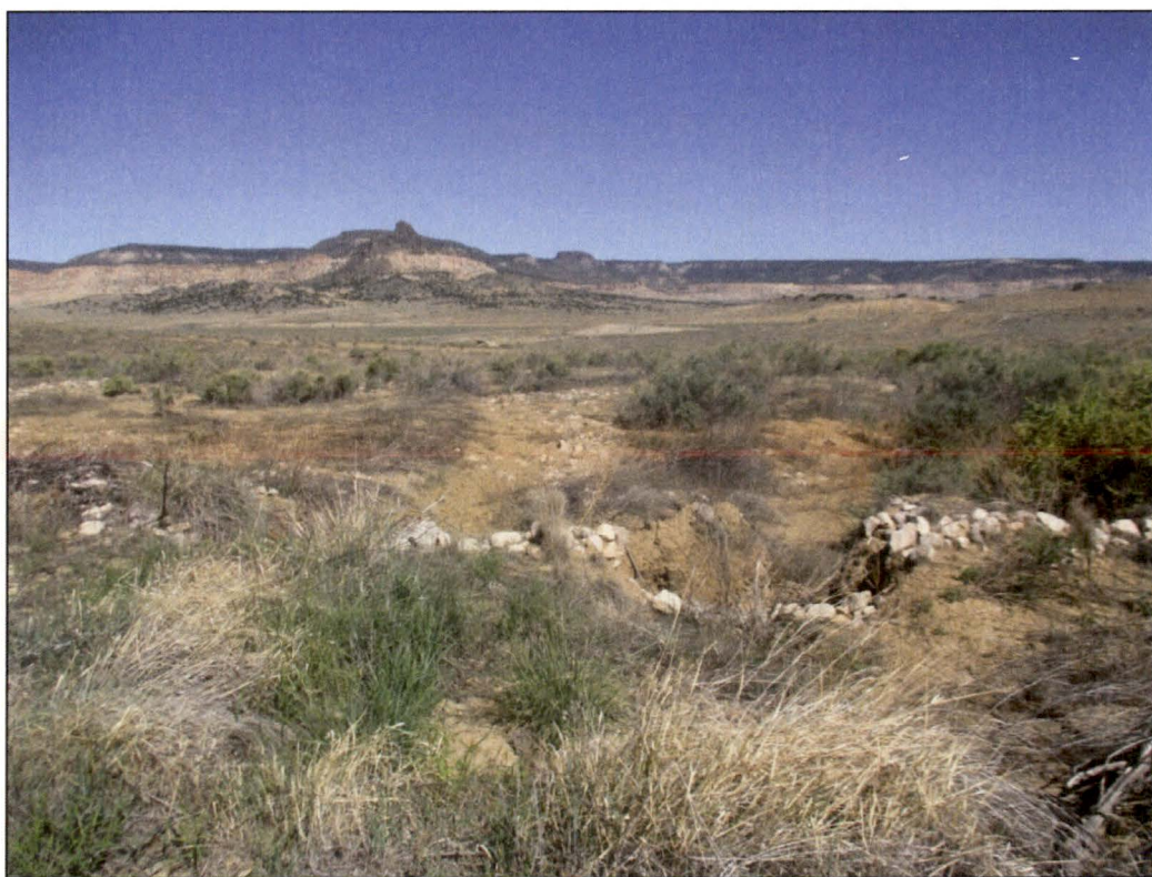
PL-12. Breach of Runoff Control Structure A Berm
