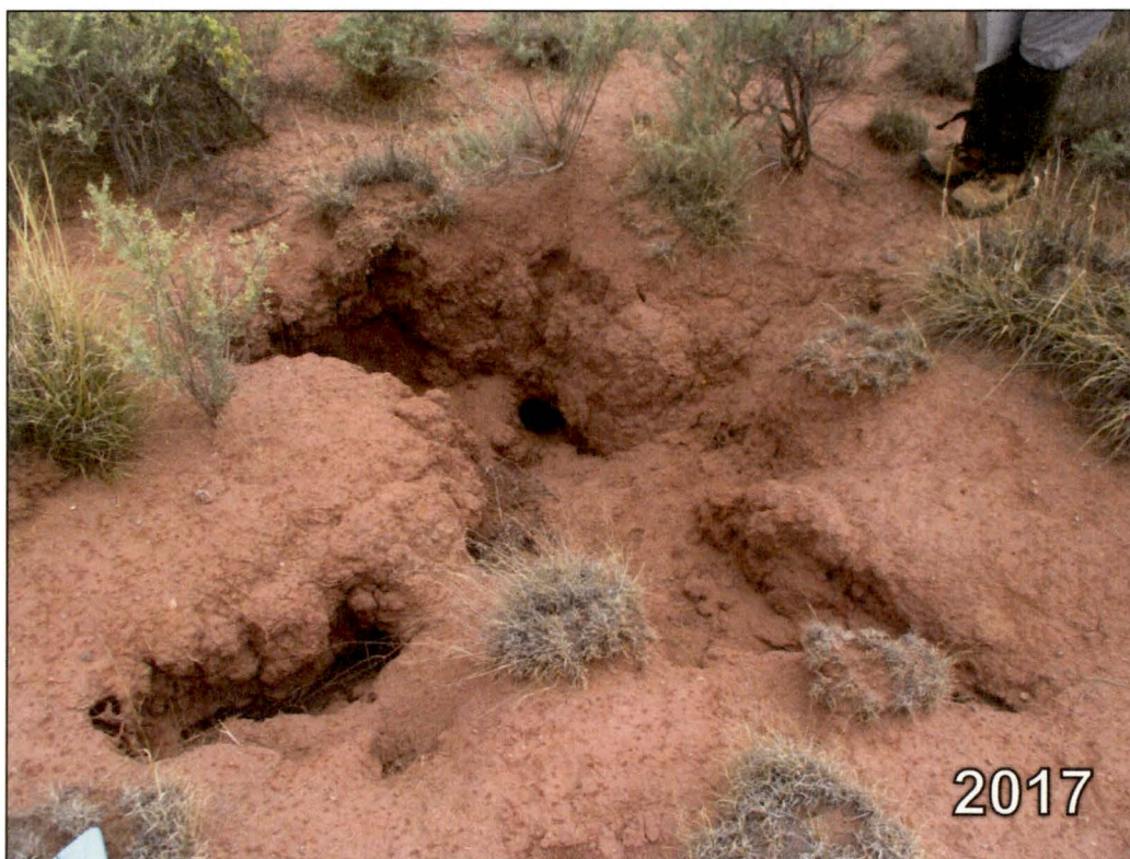
PL-17. (b) Settlement on Soil Cover of Disposal Area No. 1–2017 (Photo for Comparison)
