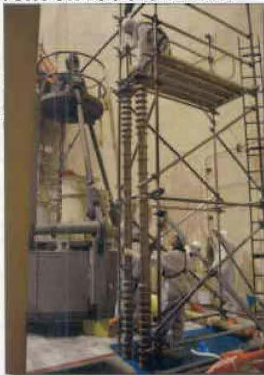
The Emergent Issues Team is working a plan to remove control rod drive mechanism coil stacks and dummy cans on spare penetrations to address the reactor head issues.
