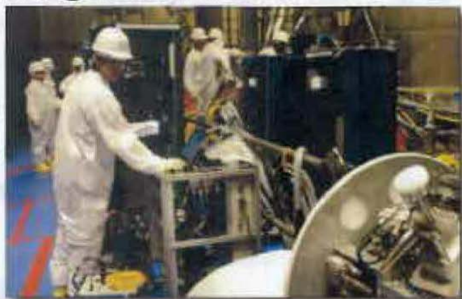
The team has worked through issues with the water jet peening tools and is now making steady progress with peening the reactor vessel and bottom nozzles.
