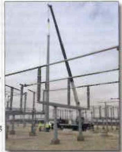
Water jet peening officially got underway yesterday morning on the "D" reactor vessel cold leg nozzle. Below, the lightning mast was installed in the switchyard last week as part of the lightning protection and grounding system changes.
