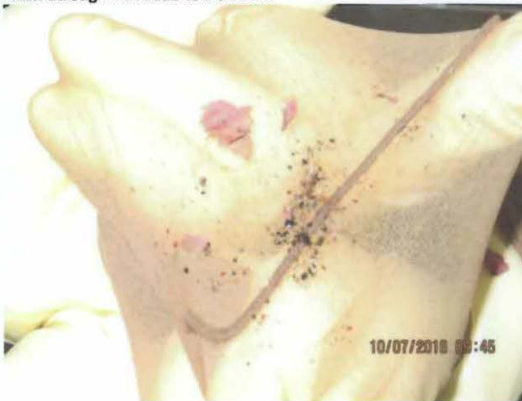
Flush through BGV0818 to BGV0459
