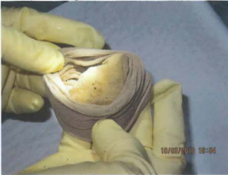
BGV0460, NCP Discharge Drain Valve
