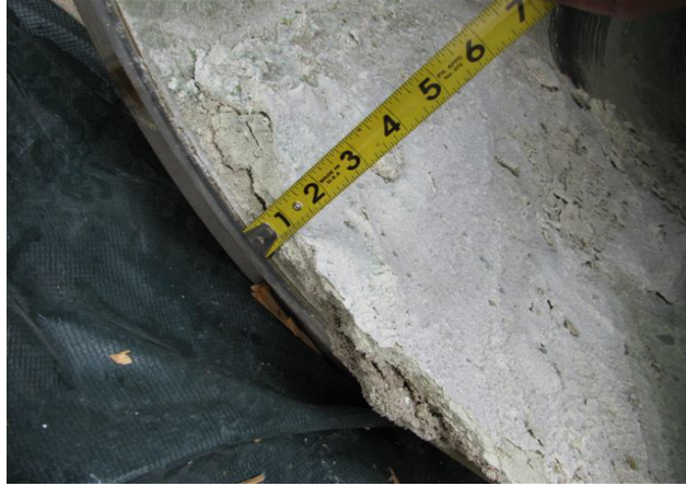
May 27, 2016 Inlet Transition Elbow
