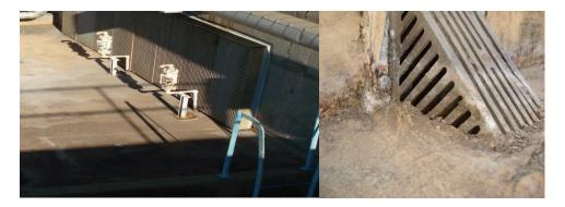
Both the train A and B vents were located on the roof of the same structure. The roof has a berm along the top of the perimeter. The photo on the right captures the scupper enclosure. All of the roof water would drain through this single drainage point. A piece of foreign material was also found on the roof. This material could block a portion of the scupper.
