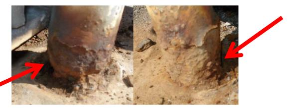
The above photos capture the thru-wall holes at the base of each 1 inch diameter vent pipe, where they exit the roof. A head-on view of the West vent hole is provided in the two pictures below. The East hole is not shown and was reported by the team as being the larger hole. An ink pen is shown in the right picture for perspective.
