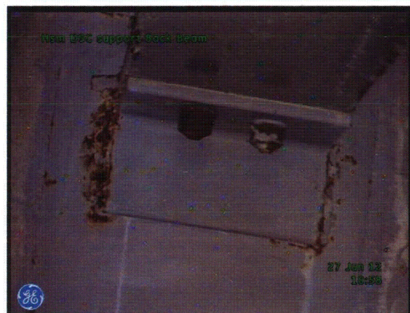
HSM-15 East Back Beam Embedment Weld
