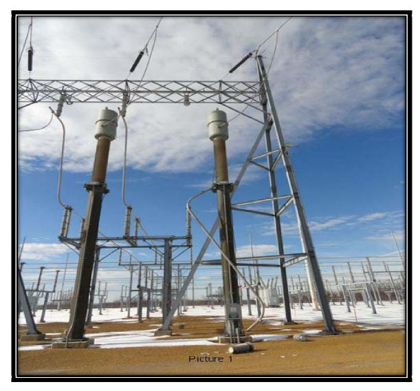
The broken insulator that was providing vertical support for the "C" phase conductor resulted in the conductor breaking and isolating the "C" phase 345kV supply to the Unit 2 SATs. This type of "open" failure did not result in a desired protective logic actuation for the SATs or switchyard ring bus. The SAT protective relays were designed to trip during a fault or overcurrent condition, neither of which occurred. The differential relays were
