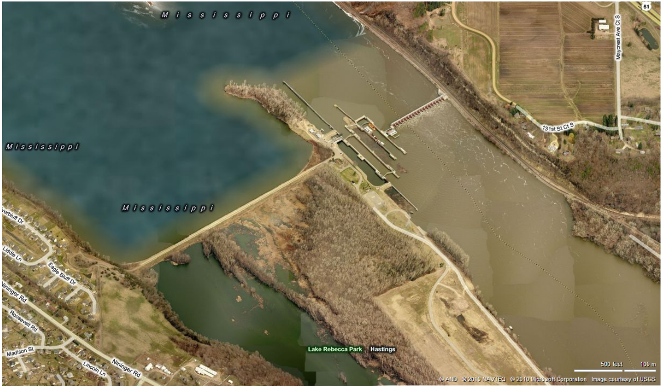
Figure 9: Aerial Photograph of Lock and Dam #2 (Earth and Concrete Sections)
