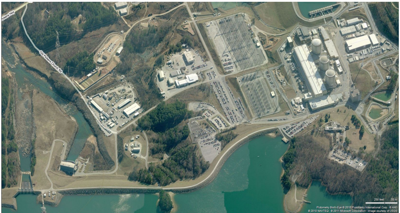
Figure 5: Aerial Photographs of Oconee Nuclear Station
