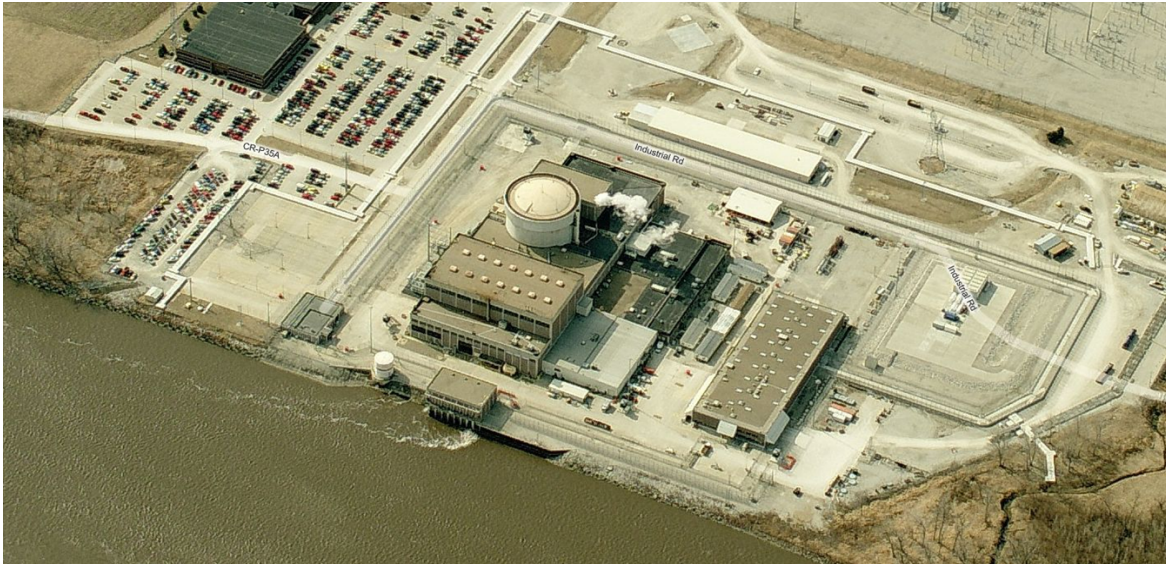
Figure 1: Aerial Photograph of Fort Calhoun Station
