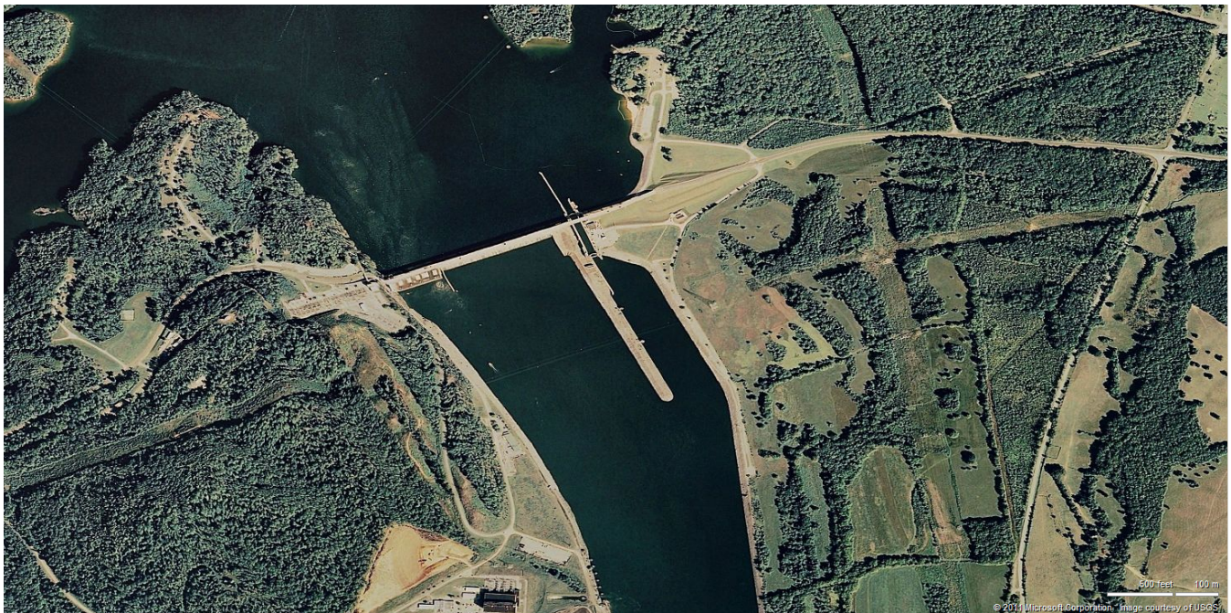
Figure 8: Aerial Photograph of Watts Bar Dam
