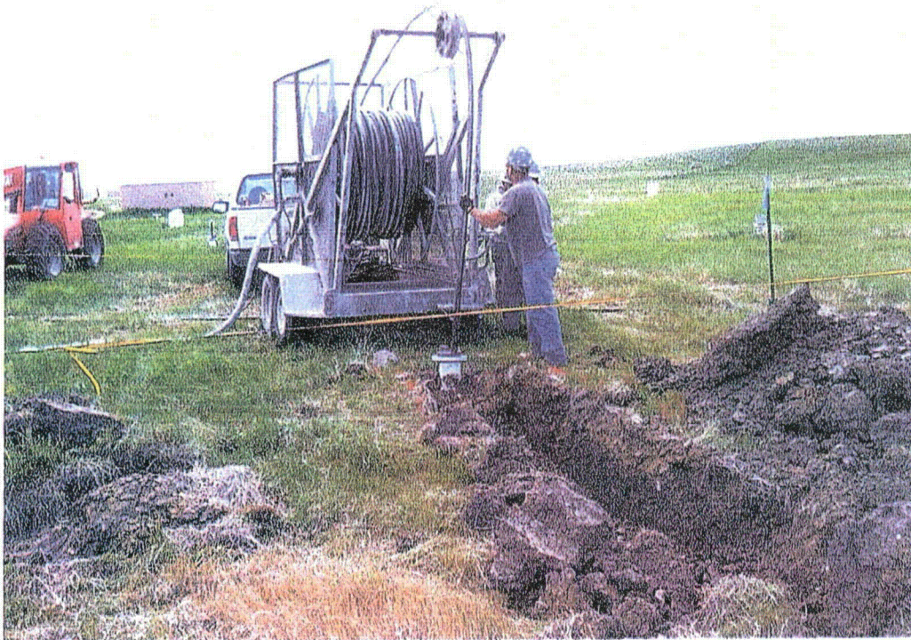
Figure 6 Hose reel and mud pit.
