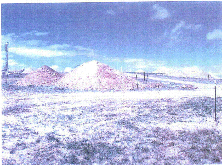
Figure 5 Mine Unit K North Development Activities without downslope erosion control
