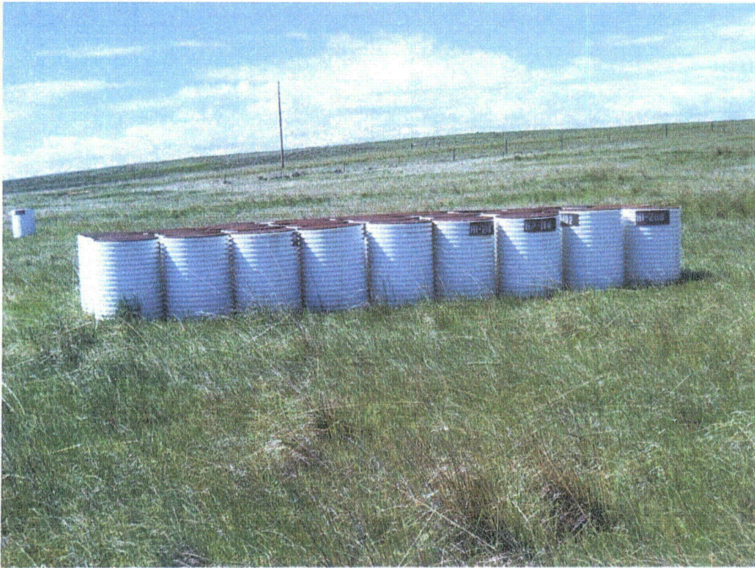
Figure 18 Well covers set along side of wellfield; not over wells
