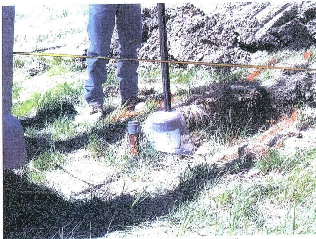
Figure 13 Pumping the cement/bentonite mixture to the bottom of the well
