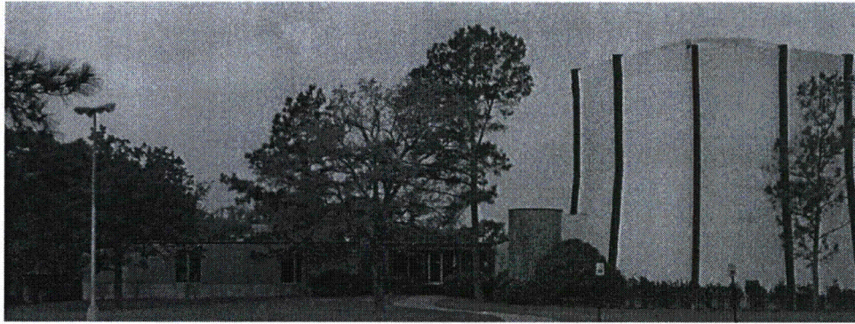
Figure 1-1: Nuclear Science Center Reactor and Laboratory Buildings
