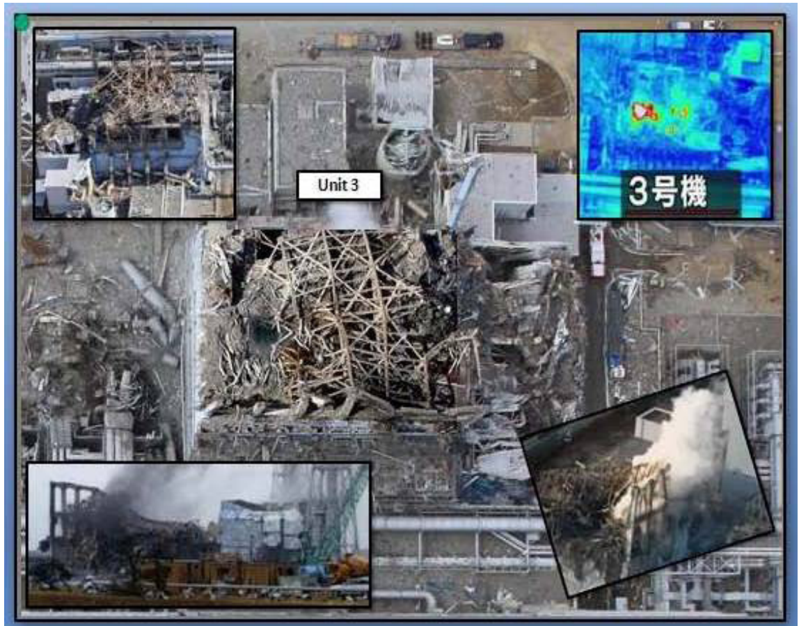
Figure 5: Damage to Unit 3
