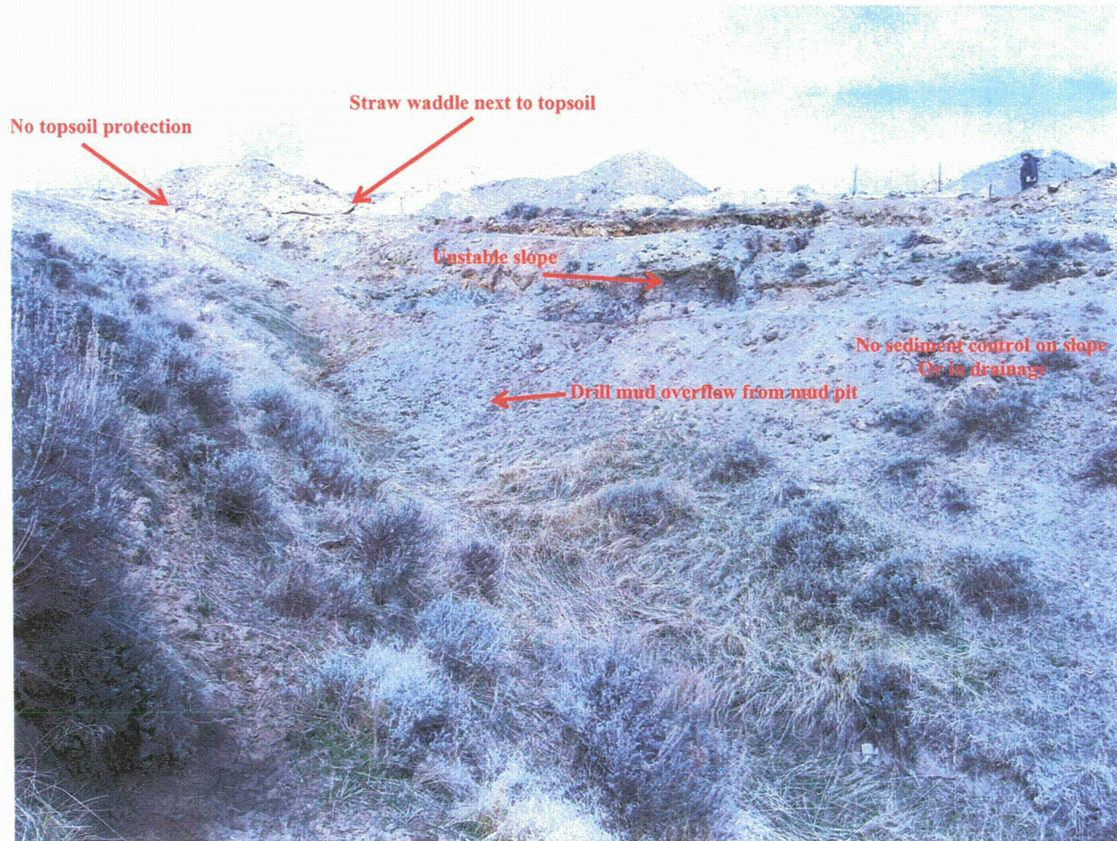
Figure 11a Drill site on slope; drill mud spilled onto native, unstable drill pad, lack of sediment control in drianage, lack of topsoil protection
