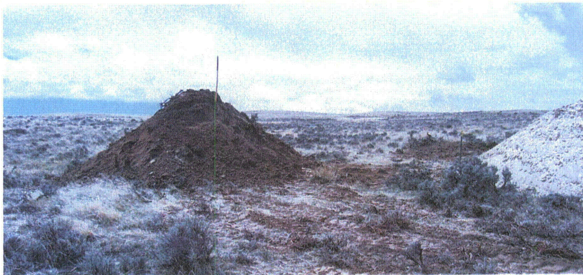
Figure 7 Topsoil pile in MU10 without erosion control
