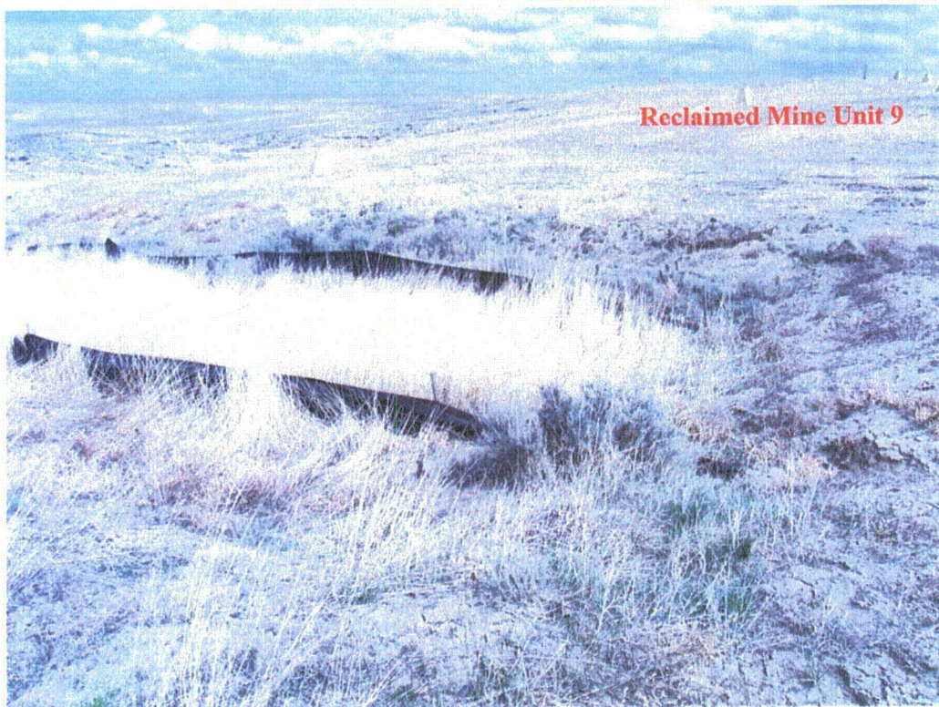
Figure 13 MU-9 temporary revegetation is completed in the wellfield (fall 2010). Sediment control is in place around the perimeter of the reclamation to protect the native areas
