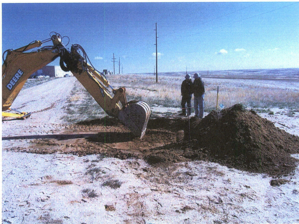
Figure 1 – Abandoned drill-hole inspection; digging to locate the drill cap
