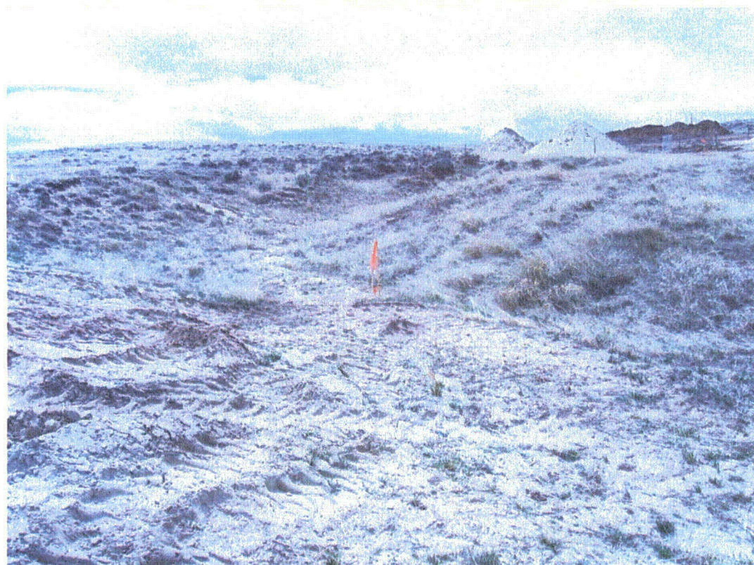
Figure 9b Disturbance in drainage without sediment control
