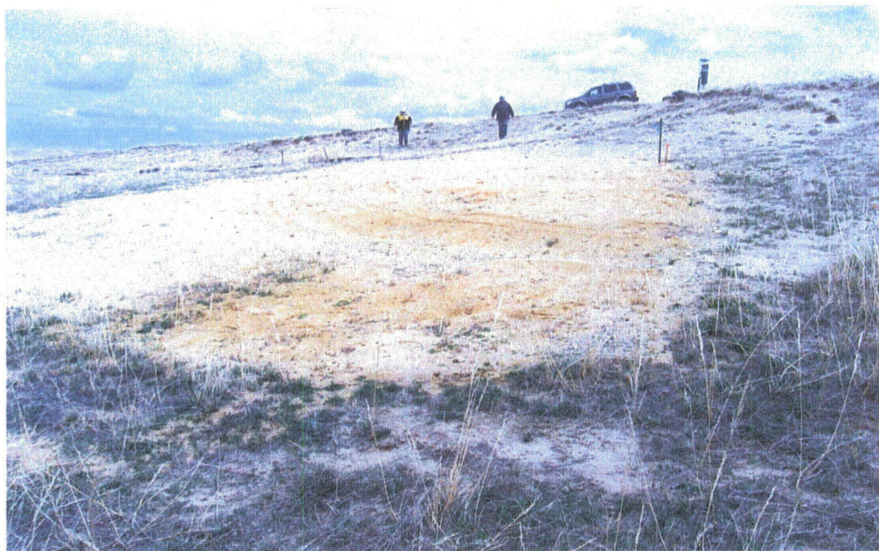
Figure 9a Disturbance area on slope without sediment control
