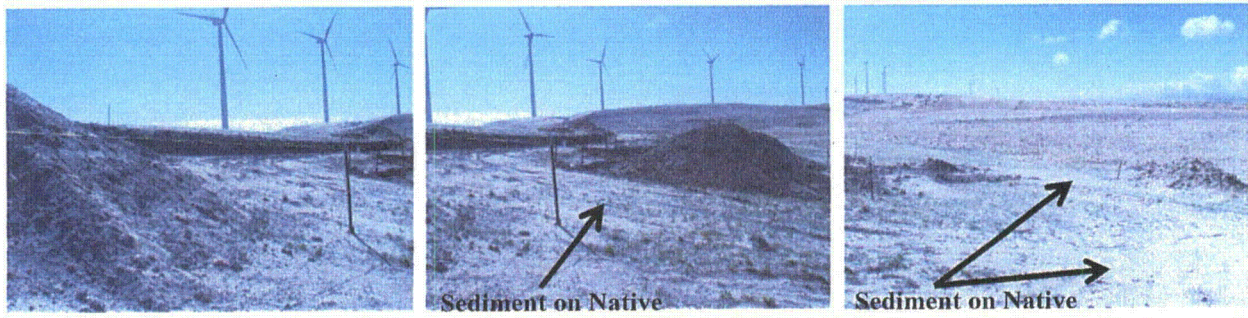
Figure 6 Drill site without sediment control resulting in sediment on native ground
