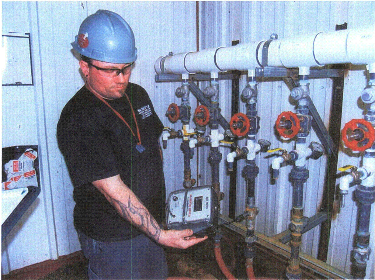
Figure 4 – Flow Meter Verification at header house
