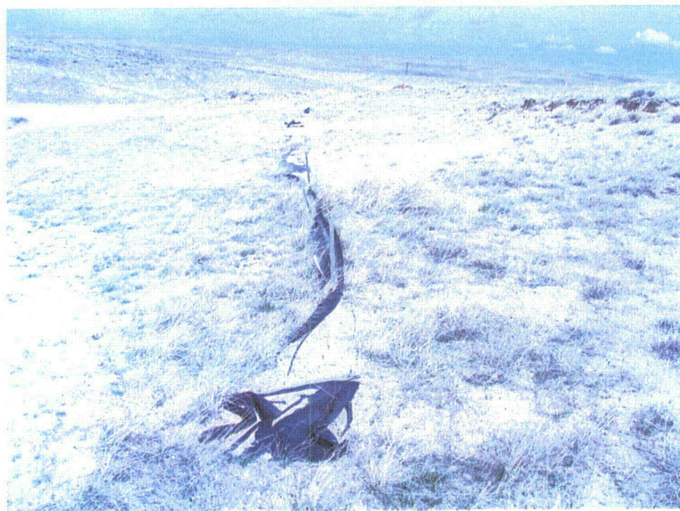
Figure 10b Poorly maintained silt fence in MU-10
