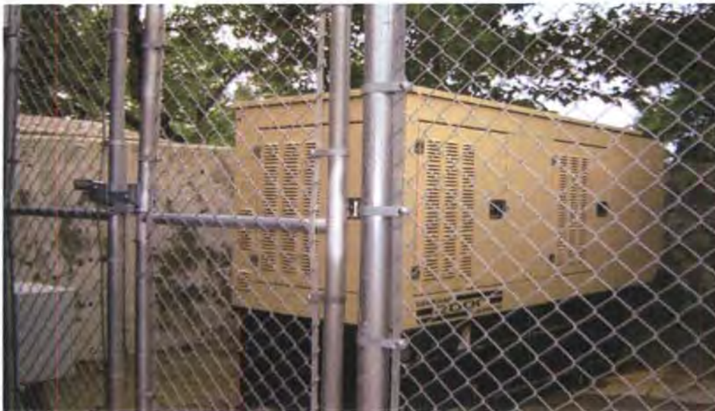
Figure 8.1-1 The control box for the electrical power system for the Merrill Engineering Building
