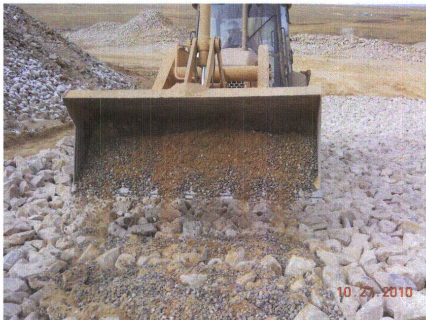
Loader spreading/sprinkling of bedding material on the surface of the riprap.
