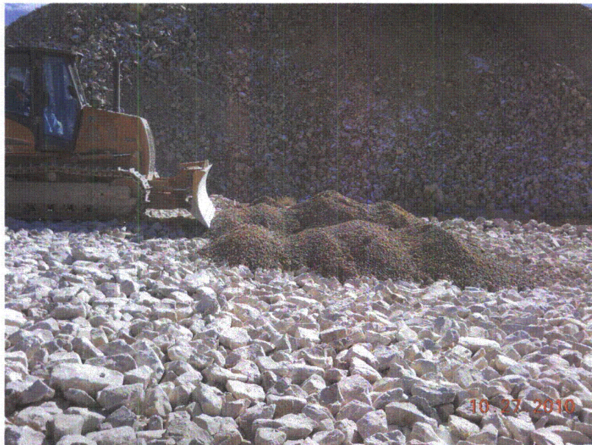
Conventional dumping of 30/70 bedding material on the surface, spread with a dozer.
