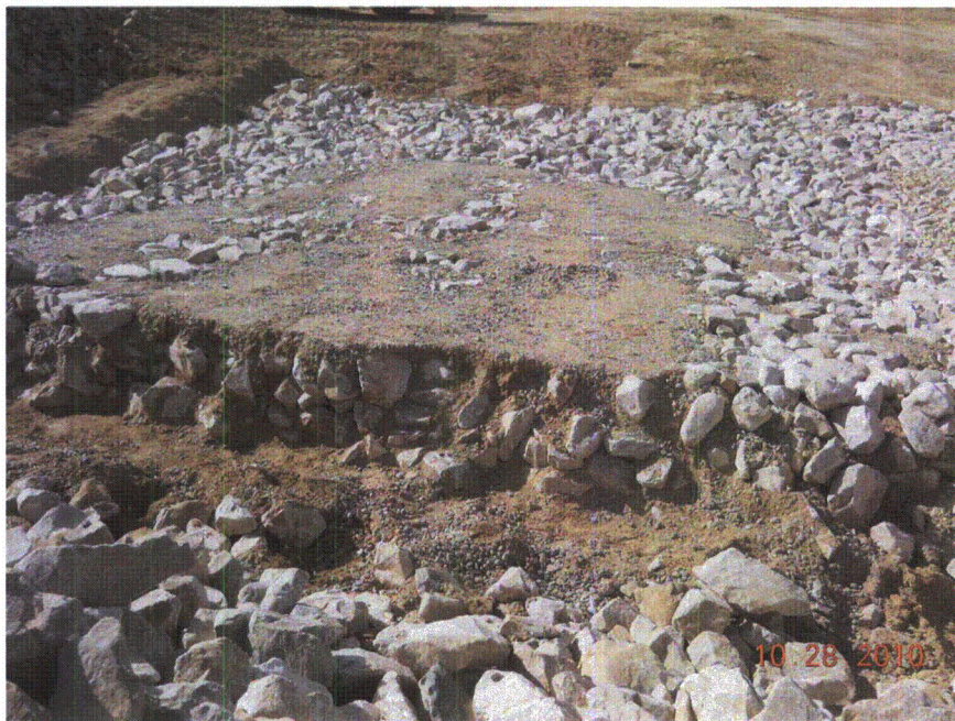
30/70 Blend bedding material placed by conventional dump/dozer spread and dozer track walked/vibrated into place. Note full penetration of bedding material in riprap layer, visible bedding material on surface and amount of waste.
