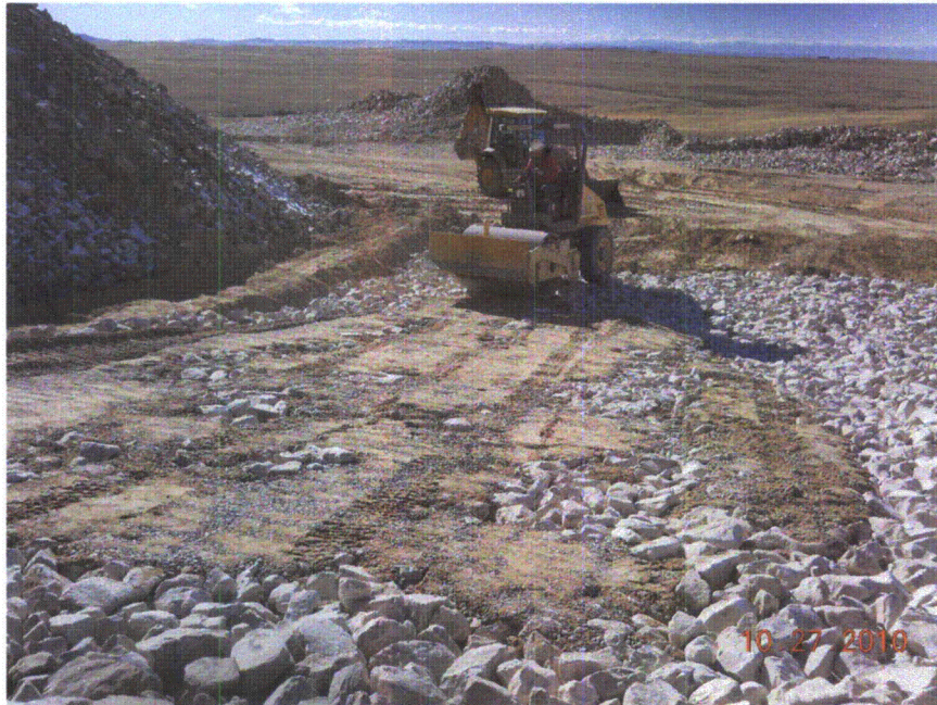
Smooth drum rolling the 30/70 blend bedding material placed by conventional methods.
