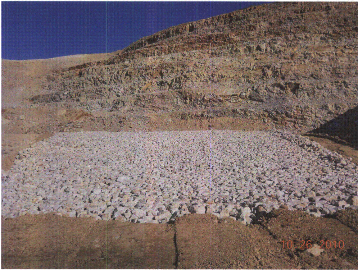
The completed Type C erosion protection material test pad.
