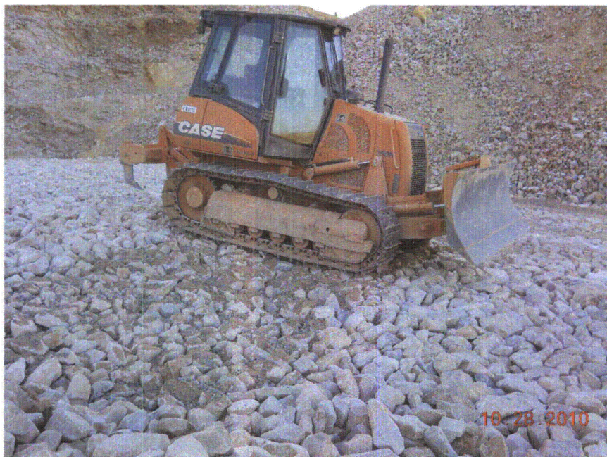
Both placement methods (loader spread and conventional dump/dozer spread), were tracked walked and rolled with a vibratory smooth drum compactor.
