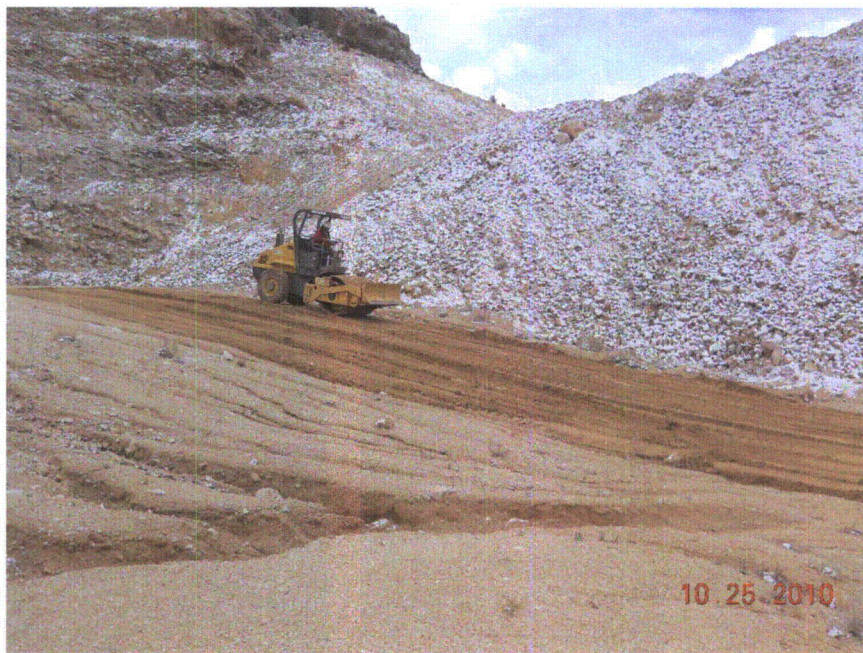
The test pad area was shaped and compacted prior to the placement of Type C erosion protection material.
