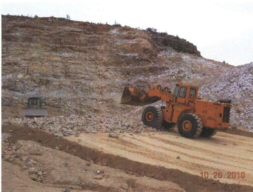
Type C erosion protection placement on the test pad slope. Riprap was placed to provide a minimum layer thickness of 12 inches.
