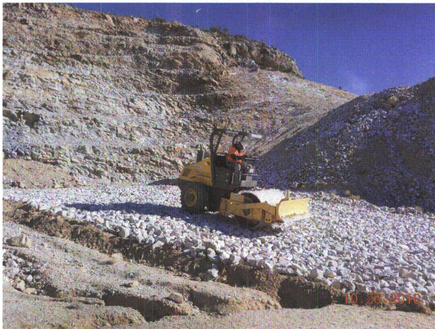
Type C erosion protection placement. Riprap was graded, tracked walked and rolled with a smooth drum compactor to duplicate the placement techniques employed on the AGTI and A-9 Repositories.
