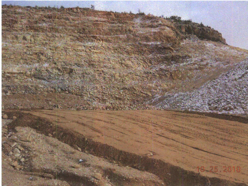
The completed sub-grade for the test pad prior to placement of Type C erosion protection material.
