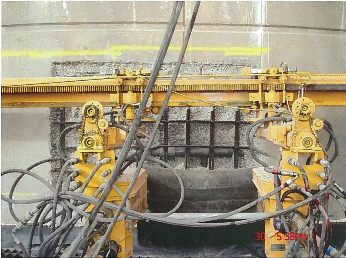
Figure A4.2 Photograph of overall status of demolition taken on 9/30/09.at 17:38
